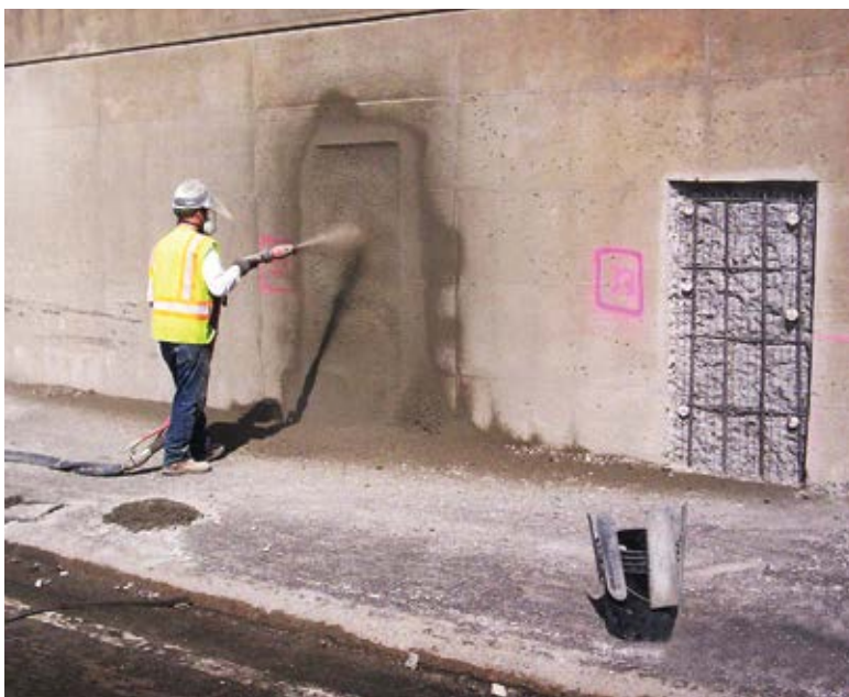
Fig. 1: Concrete (shotcrete) pneumatically projected at high velocity to repair area
