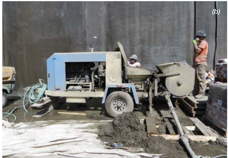
Fig. 2: (a) Dry process shotcrete gun versus (b) wet process shotcrete pump
