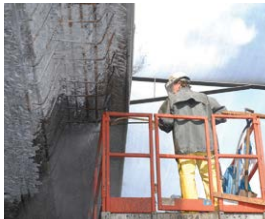
Fig. 3: High-pressure cleaning of the prepared concrete substrate prior to shotcrete application
