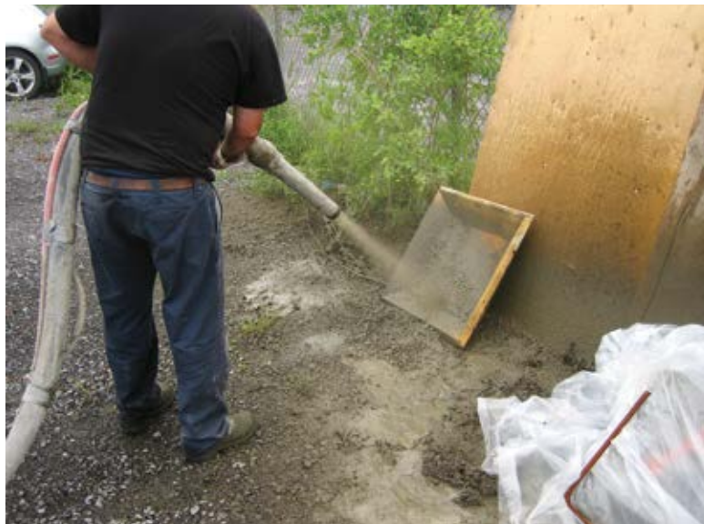
Fig. 6: Preconstruction testing of shotcrete using a test panel
