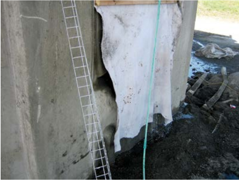
Fig. 5: Curing a vertical shotcrete repair area using a curing blanket
