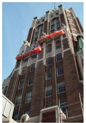
Fig. 7: Swing staging with larger work platforms and ability to capture debris
