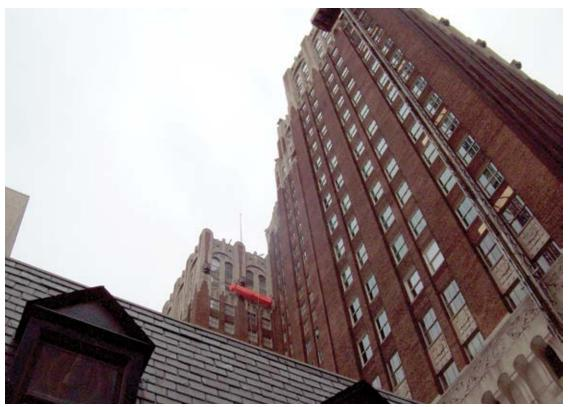
Fig. 4: Multiple access methods used: swing stage on left and mast climber on right
