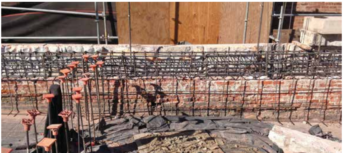
Fig. 6: Bond beam reinforcement
