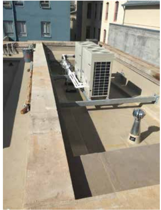
Fig. 11: Completed concrete roof work
