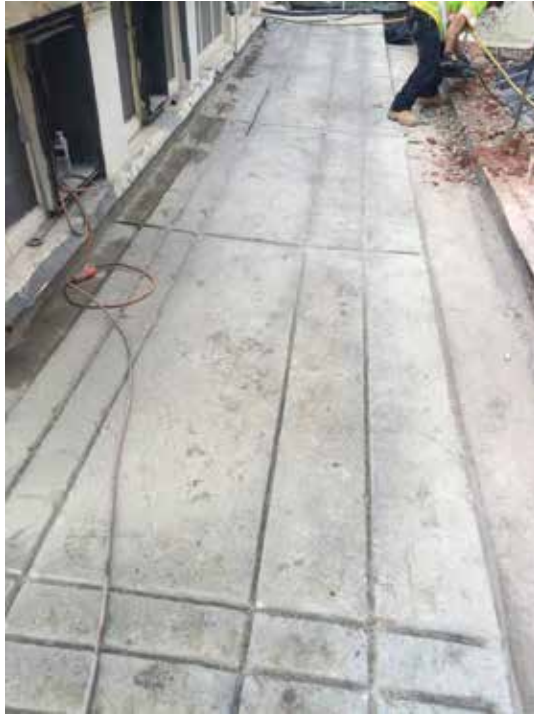
Fig. 7: NSM CFRP geometry
