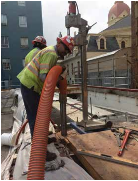
Fig. 5: Center core drilling
