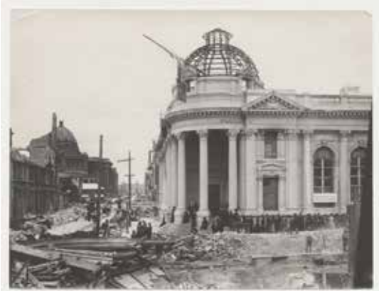
Fig. 1: Hibernia Bank after 1906 earthquake
