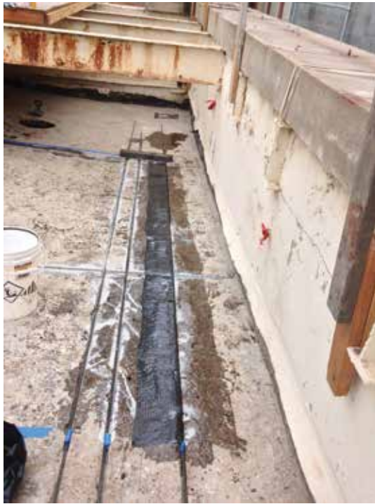
Fig. 9: FRP starter sheet application
