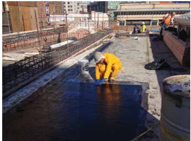
Fig. 10: Roof FRP installation
