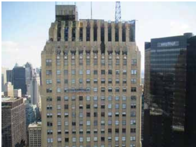
Fig. 8: View of the east elevation with the southeast corner completed and the southwest corner not started
