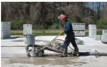
The live demo included a hydrodemolition machine...
