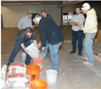
Hands-on training included working directly with some concrete repair products
