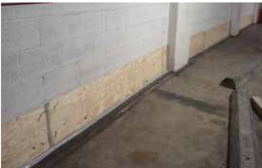
Fig. 4: Sealed skirt dam installed at perimeter of work area
