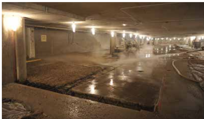
Fig. 1: Hydrodemolition of a garage floor slab
