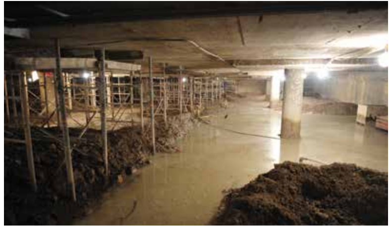
Fig. 3: Hydrodemolition waste water must be collected, settled, filtered, and treated
