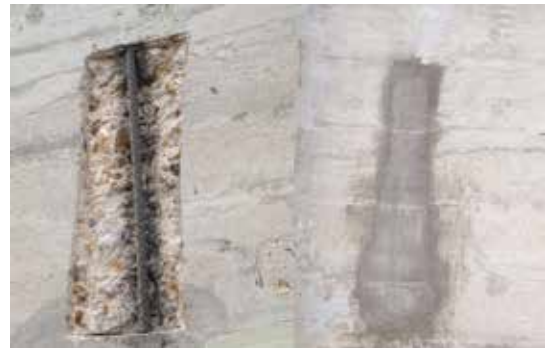
Fig. 7: Concrete spall repair
