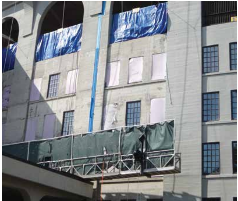
Fig. 9: Dust and overspray protection at façade
