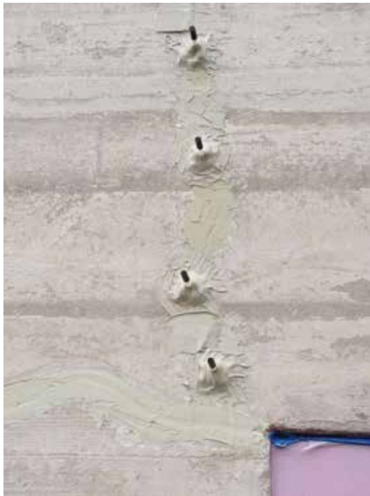
Fig. 6: Epoxy crack injection surface seal and ports
