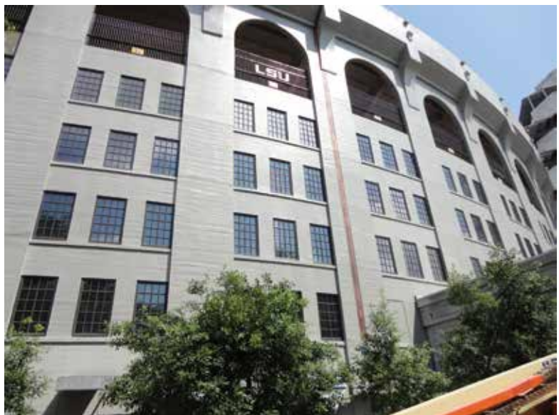
Fig. 10: Completed restoration at north end of stadium
