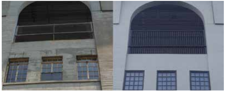
Fig. 8: Façade coating (before and after)
