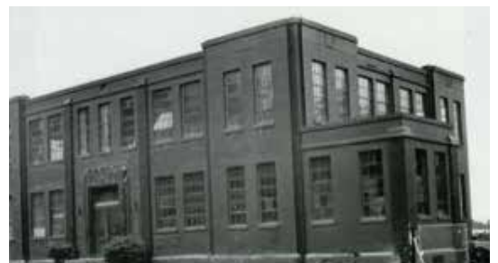
Fig. 3: Archival photograph of Sage Memorial Building with ornamental parapet removed, likely 1960s (Sitka Historical Society)
