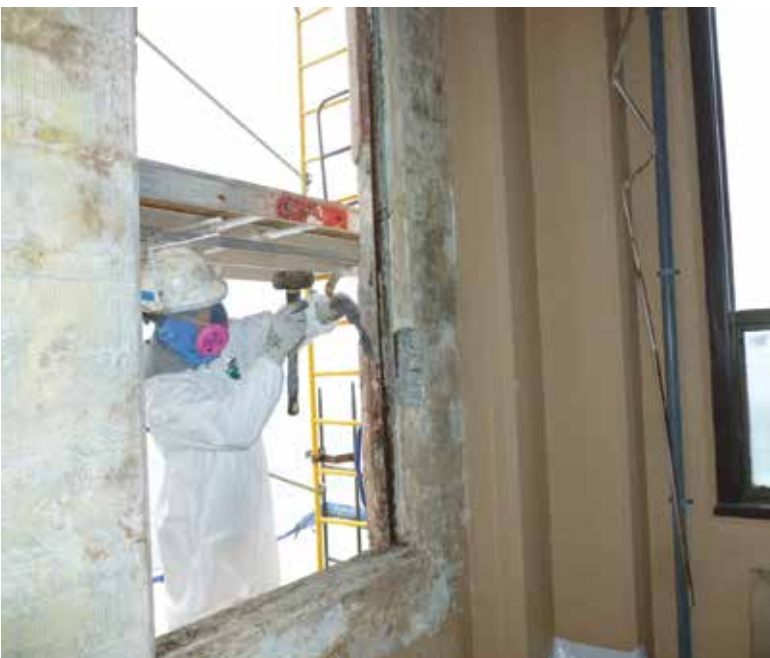
Fig. 7: Removal of steel frame embedded in concrete at window opening (2014)
