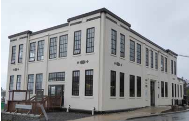
Fig. 10: Completed repair and rehabilitation of exterior concrete facade (2015)
