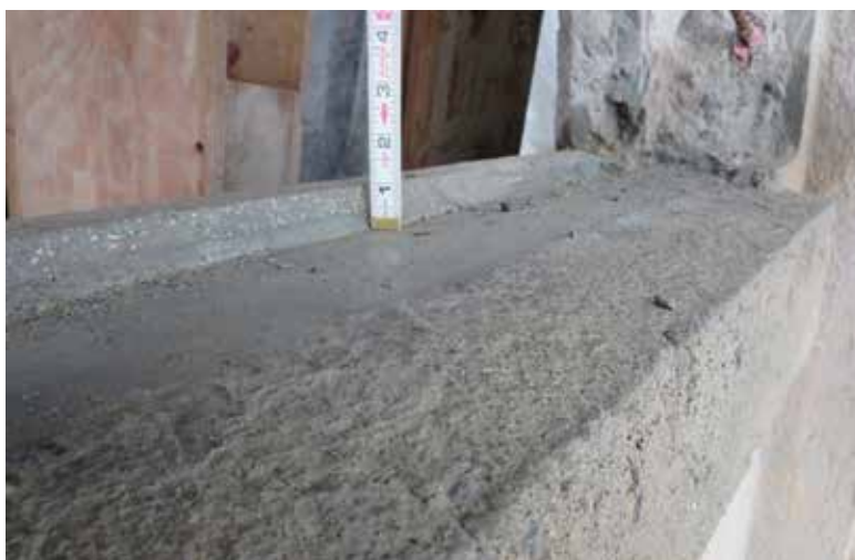
Fig. 9: Modified concrete window sill with recessed flashing ledge (2014)
