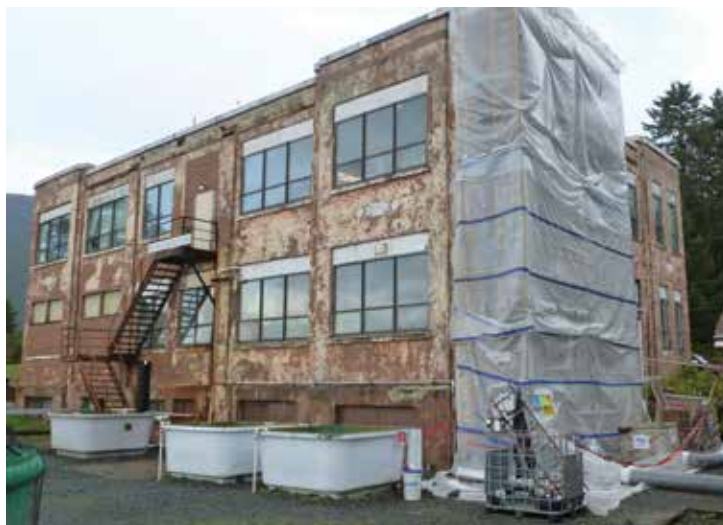
Fig. 4: South elevation facing Crescent Bay prior to repairs, during mock-up phase (2014)
