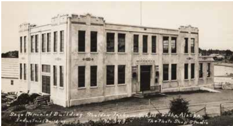
Fig. 1: Archival photograph of Sage Memorial Building with ornamental parapet (1935, Sitka Historical Society)
