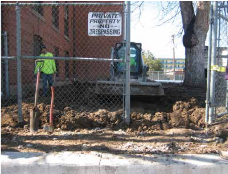
Fig. 4: Sidewalk replacement on north side of building
