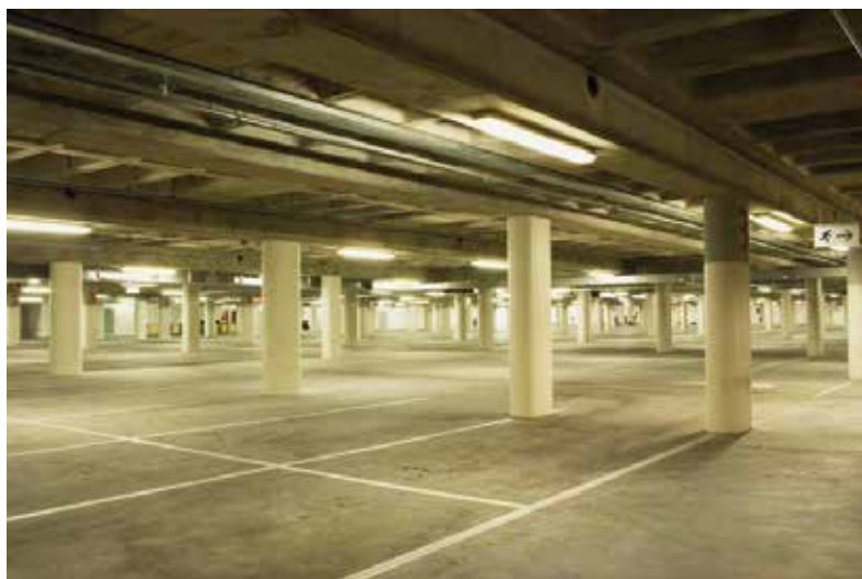
Fig. 1: Typical parking garage
