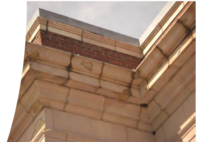
Joint Failure
