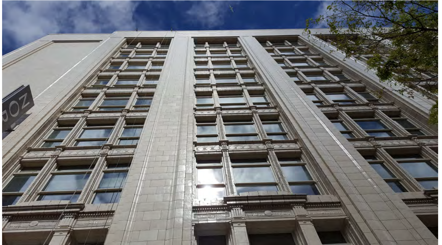
Nordstrom Flagship Store Seattle
