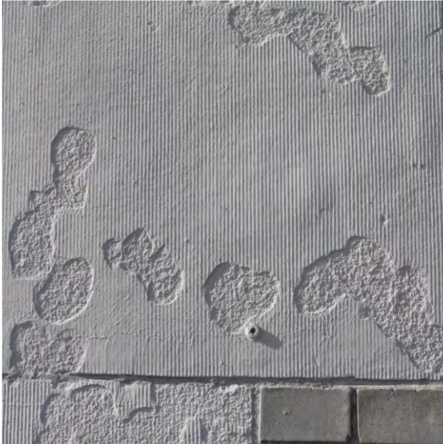
Coating Over Glaze Spalls Without Patching
