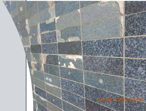
Glaze Spalling
