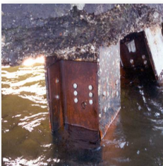
»Corroded steel section replaced with new structural steel
