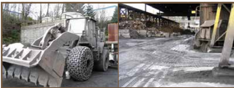
Fig. 5: Iron aggregate topping for thermal shock
