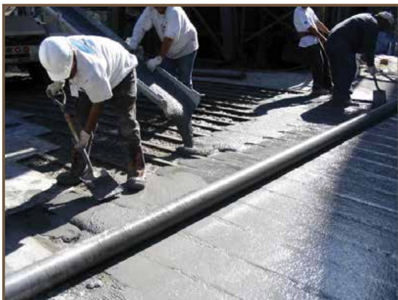
Fig. 1: The problem with railroad rails and the solution with iron aggregate topping
