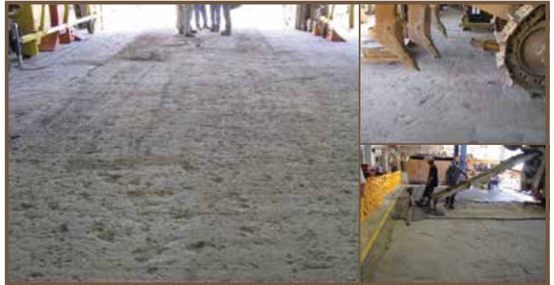
Fig. 3: Tracked vehicle maintenance bay and iron aggregate topping
