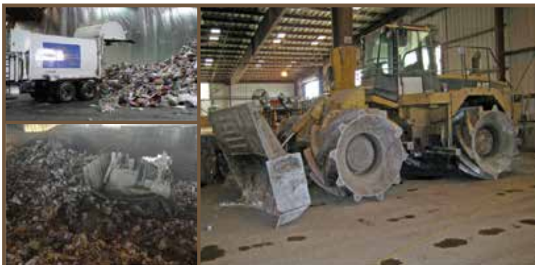
Fig. 6: Solid waste transfer station tipping floor—impact and point loads, abrasion, and chemical attack
