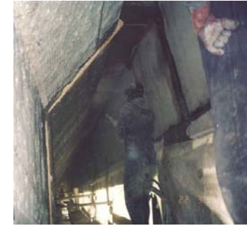
Dry sprayed overlay being applied
