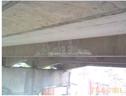
Holding repair after 9 years
