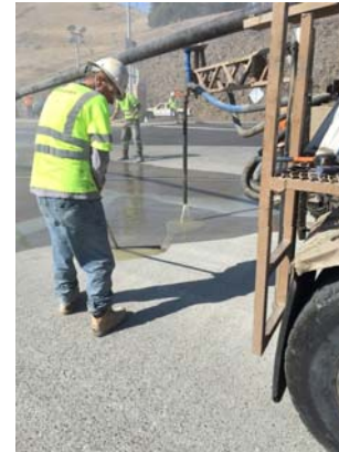
Application of epoxy
