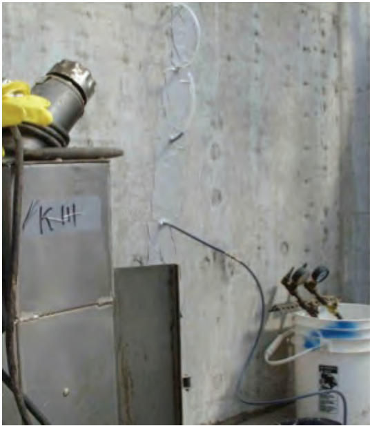
Fig. 1: Injection showing port-to-port adhesive travel
