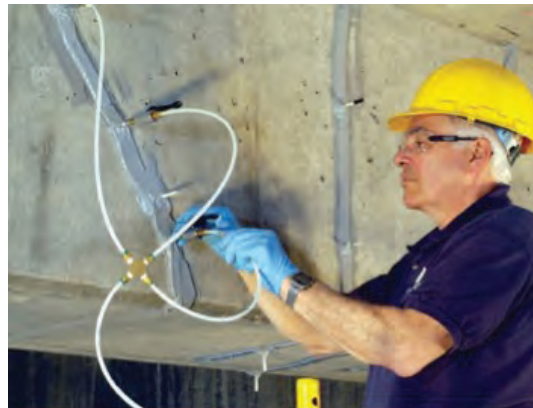
Fig. 3: Injection using a manifold system
