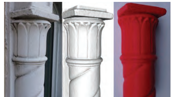
Fig. 6: Left - Existing decorative column, Middle - 3D model of column, Right - 3D print of model
