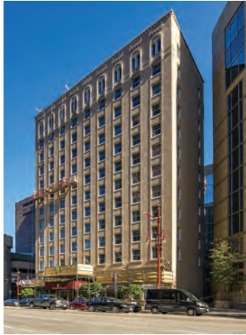
Fig. 12: Contractor performing repairs on south elevation of the Lan- caster Hotel
