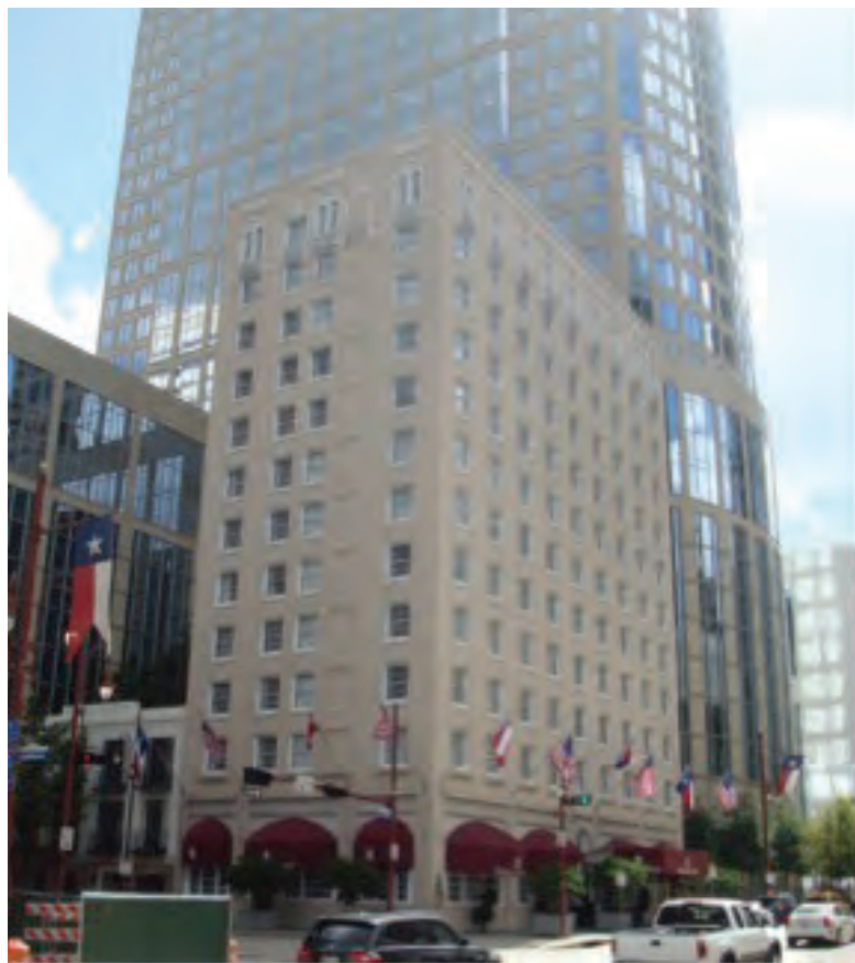
Fig. 1: Overall view of Lancaster Hotel in foreground
