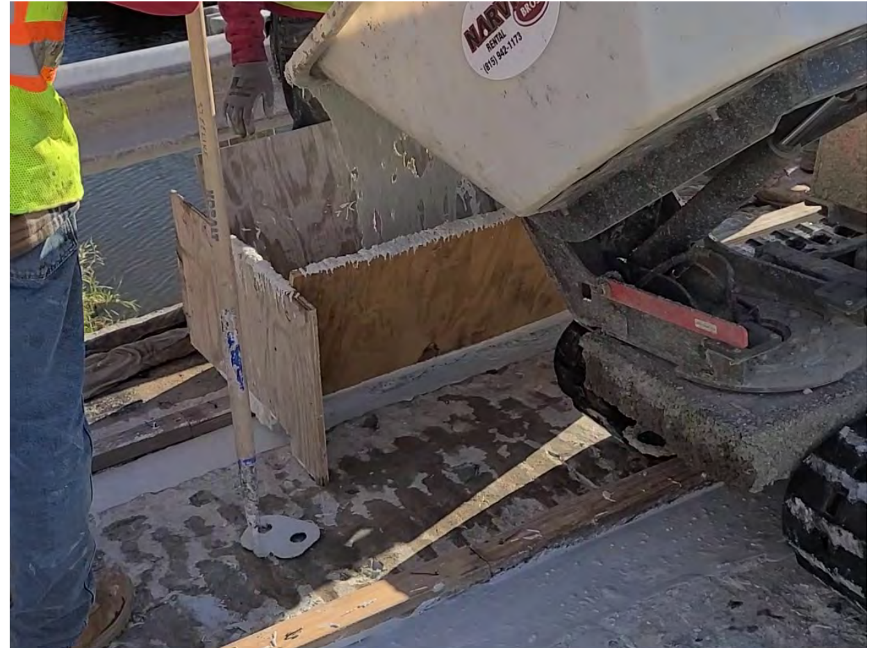
Placing UHPC in longitudinal connections with no top forms
