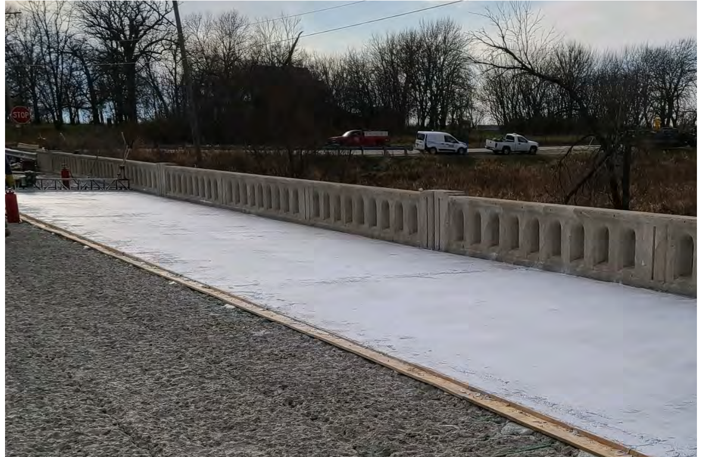
Curing UHPC overlay without plastic sheeting.
