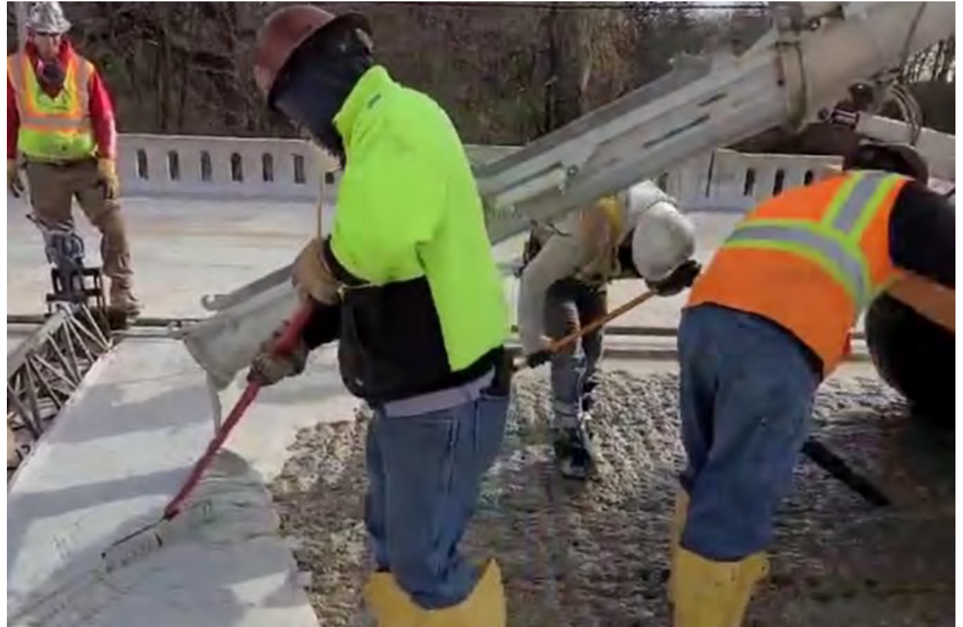
Directly discharging UHPC onto bridge deck in front of screed.
