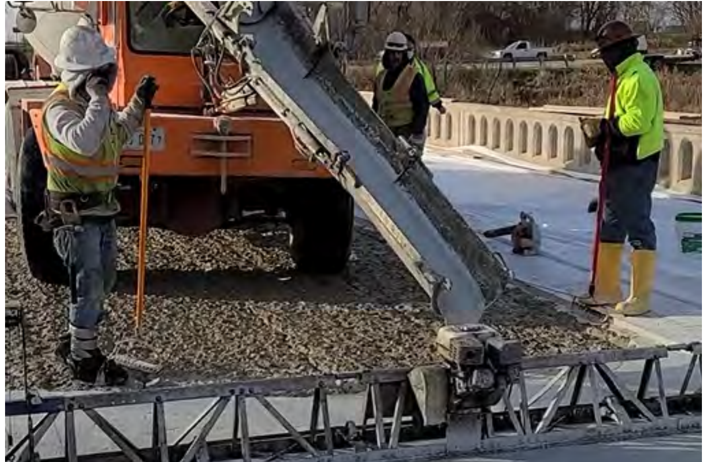
Discharging UHPC directly from ready-mix truck
