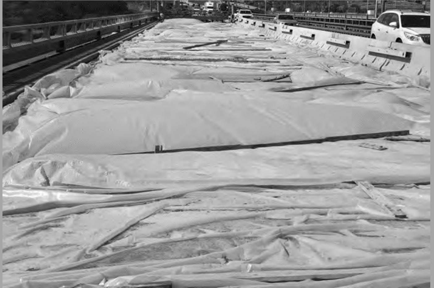
Plastic sheeting over UHPC overlay with wind blowing underneath
