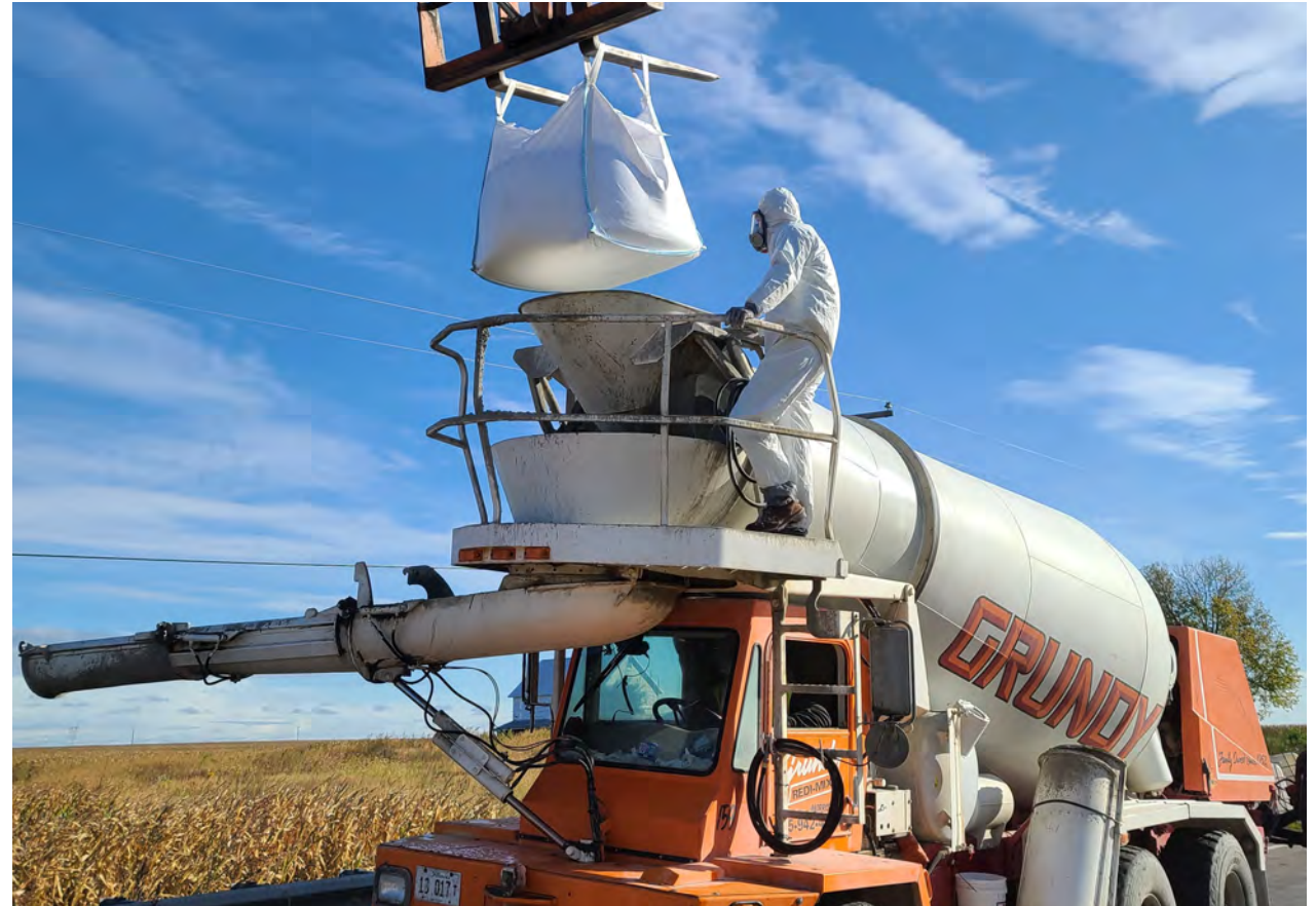
Mixing UHPC in standard ready-mix truck
