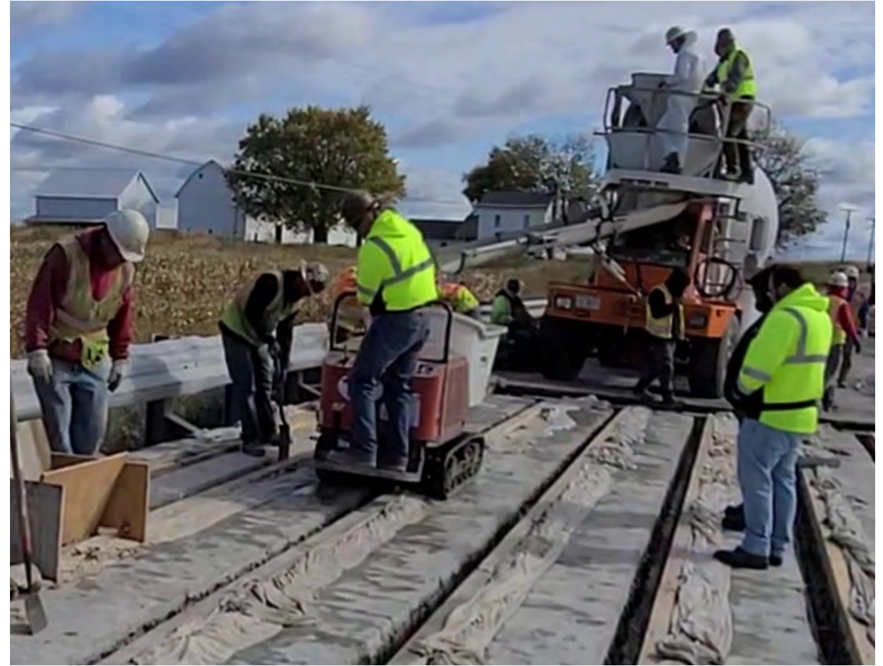
Delivering UHPC in standard ready-mix truck
