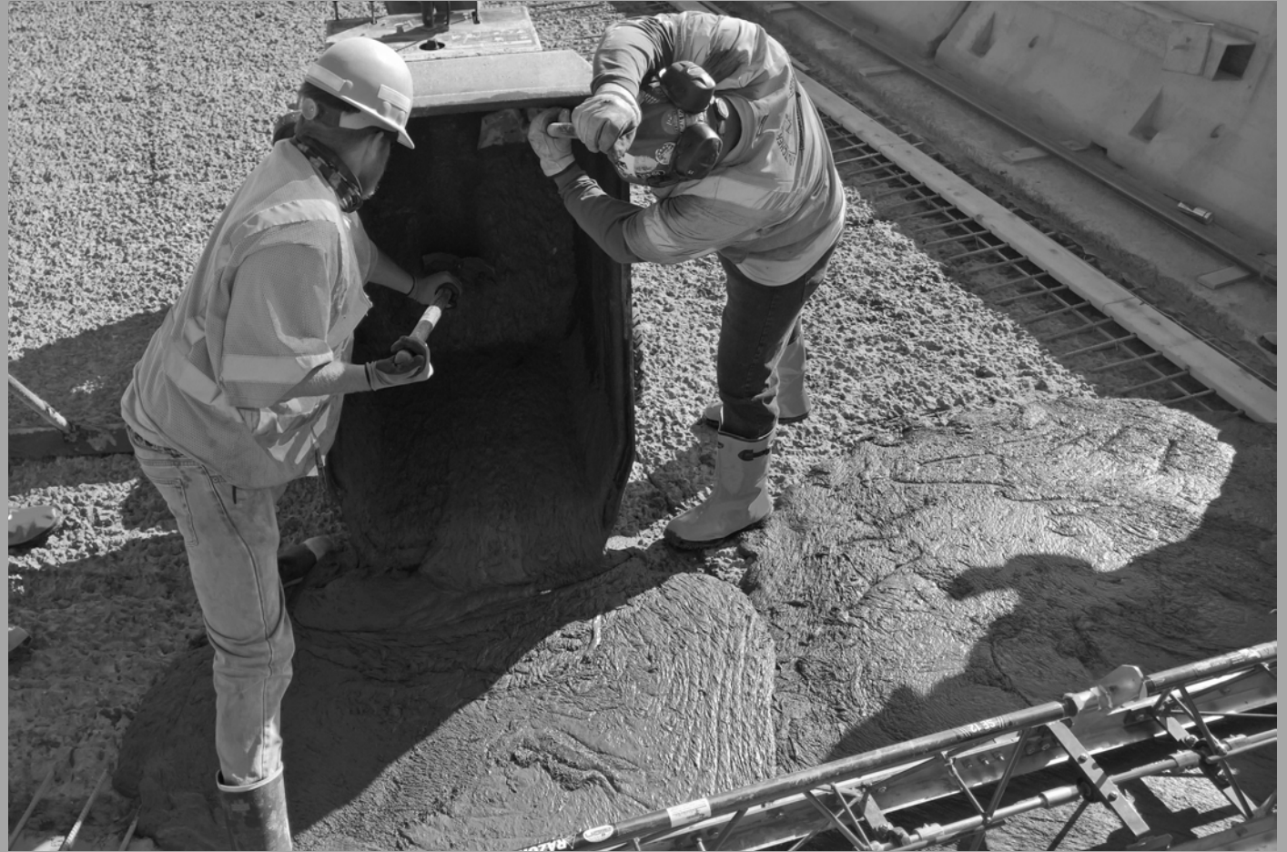
Discharging UHPC from concrete buggy in front of overlay screed
