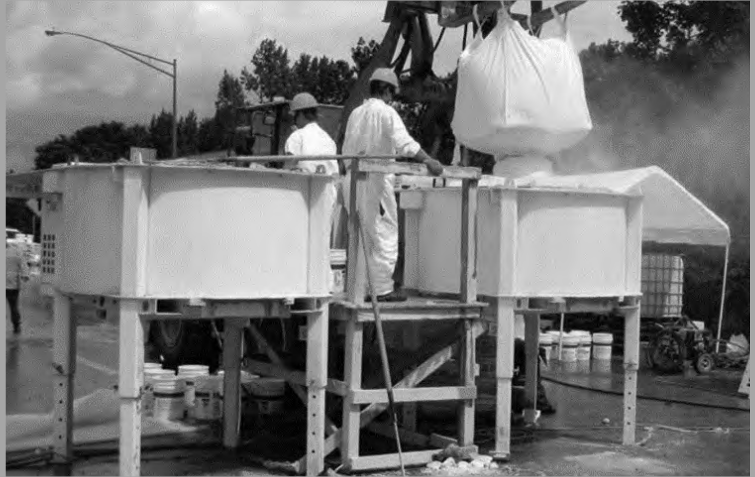
Vertical shaft high-shear mixers
