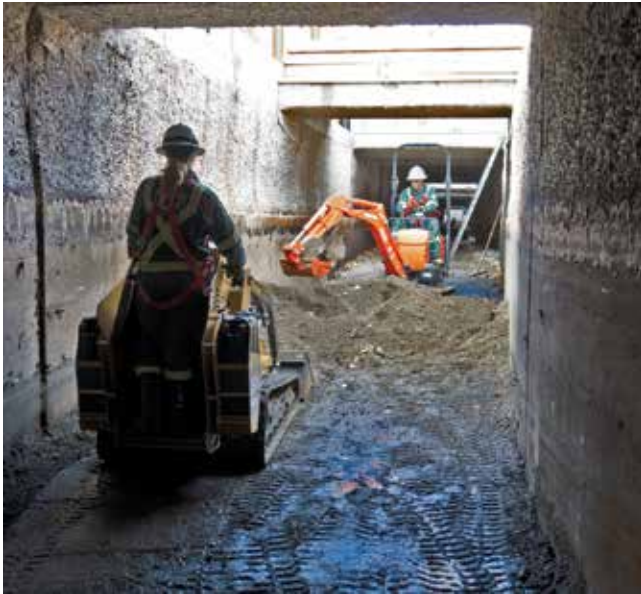
Fig. 5: Initial removal of channel debris
