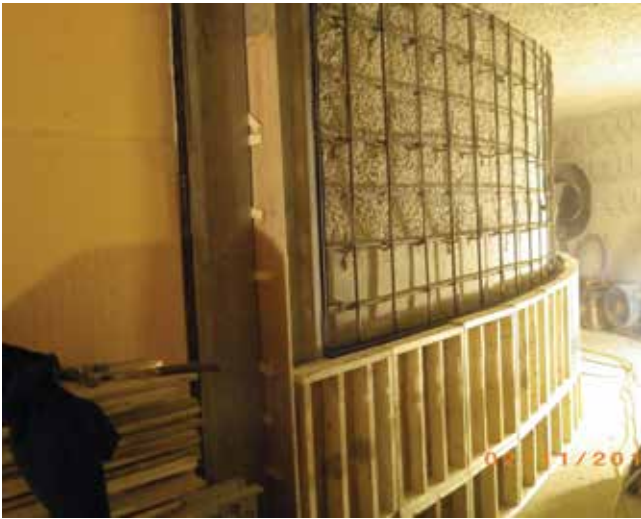
Fig. 11: Wall liner, reinforcement, and formwork
