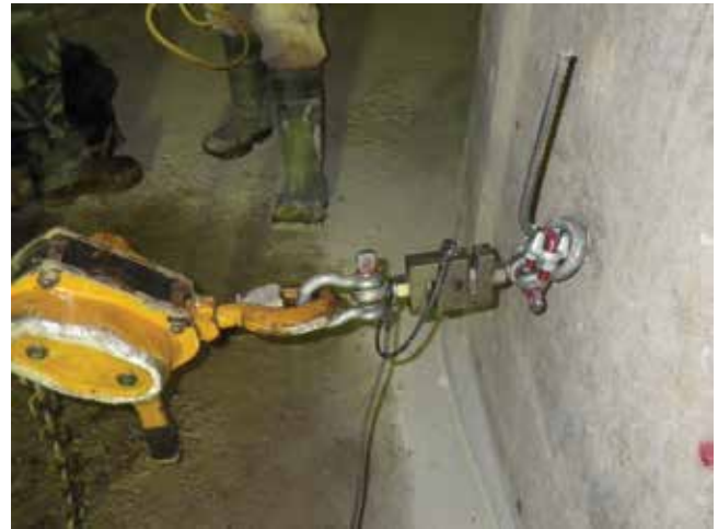
Fig. 16: Load testing of dowels
