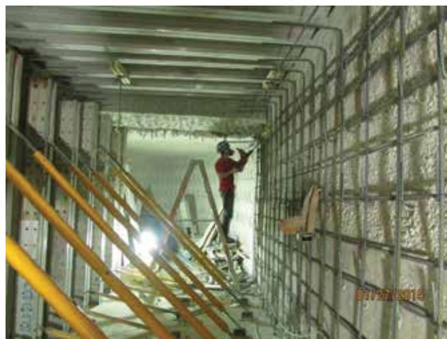
Fig. 10: Overlay reinforcement at overflow wier
