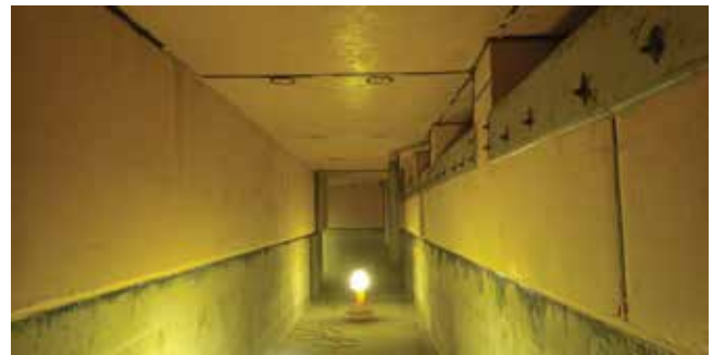
Fig. 17: Nearing completion of overlay and HDPE liner assembly at overflow wier
