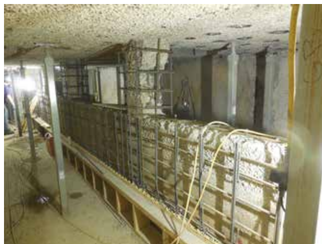
Fig. 9: Formwork, bracing and drilling of reinforcing dowels
