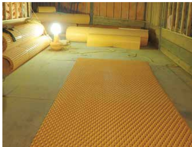
Fig. 8: Preparation of HDPE liner for installation
