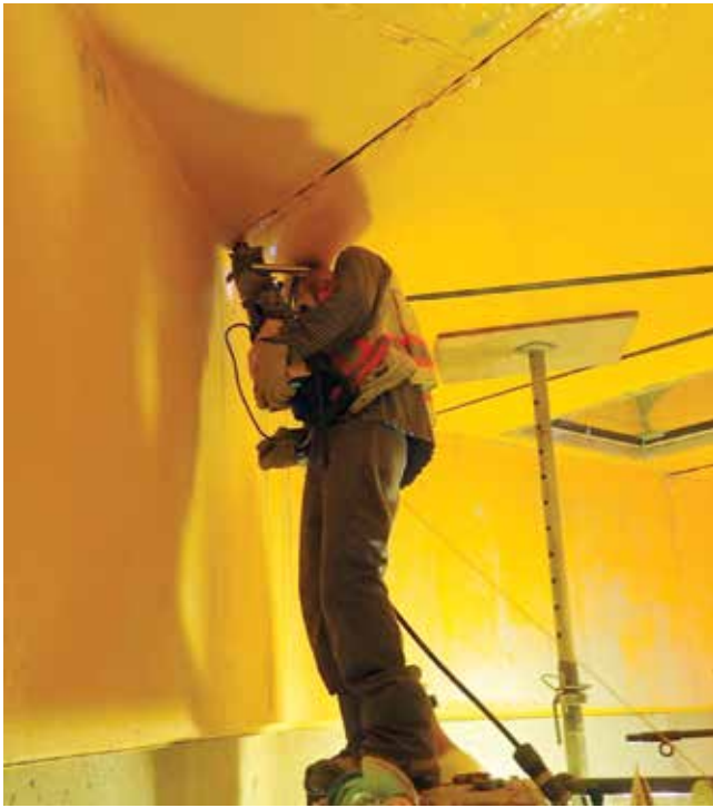
Fig. 14: Field welding of HDPE liner seams
