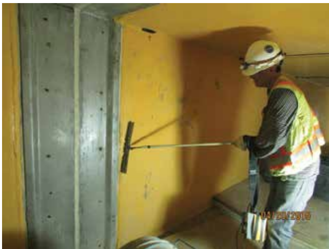
Fig. 15: Spark testing of completed HDPE liner welds
