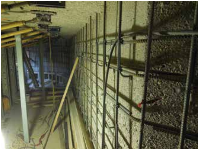
Fig. 6: Wall reinforcing and bracing
