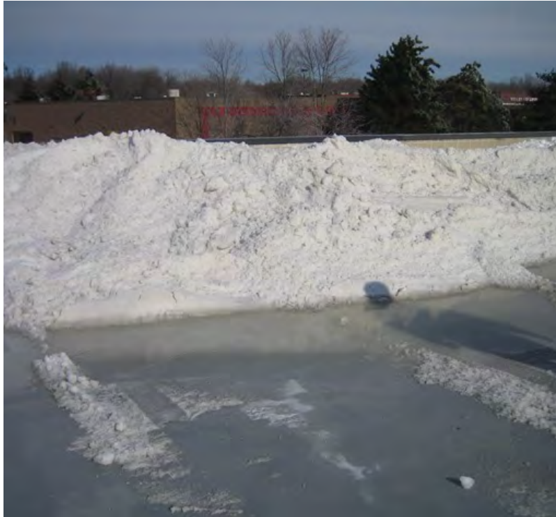
~6' Deep pile 20' wide across back of garage
