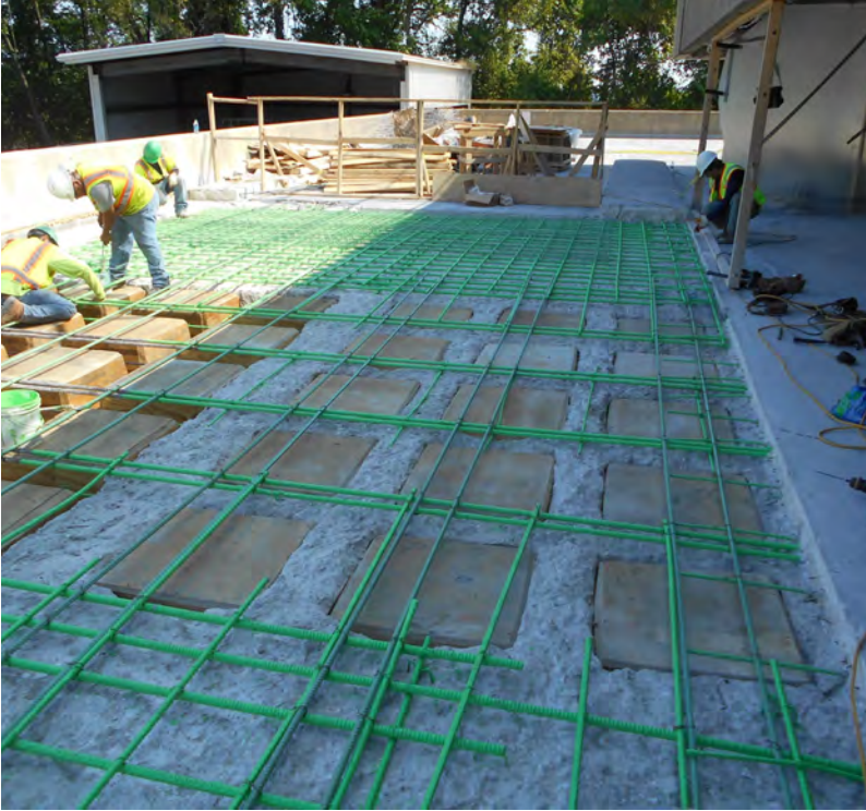
Waffle slab replacement
