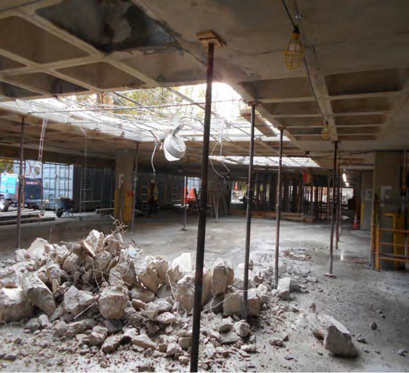
Demolition of waffle slab system
