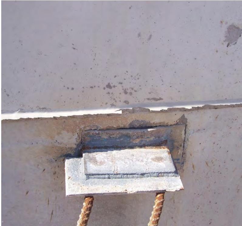
Reused existing connections
