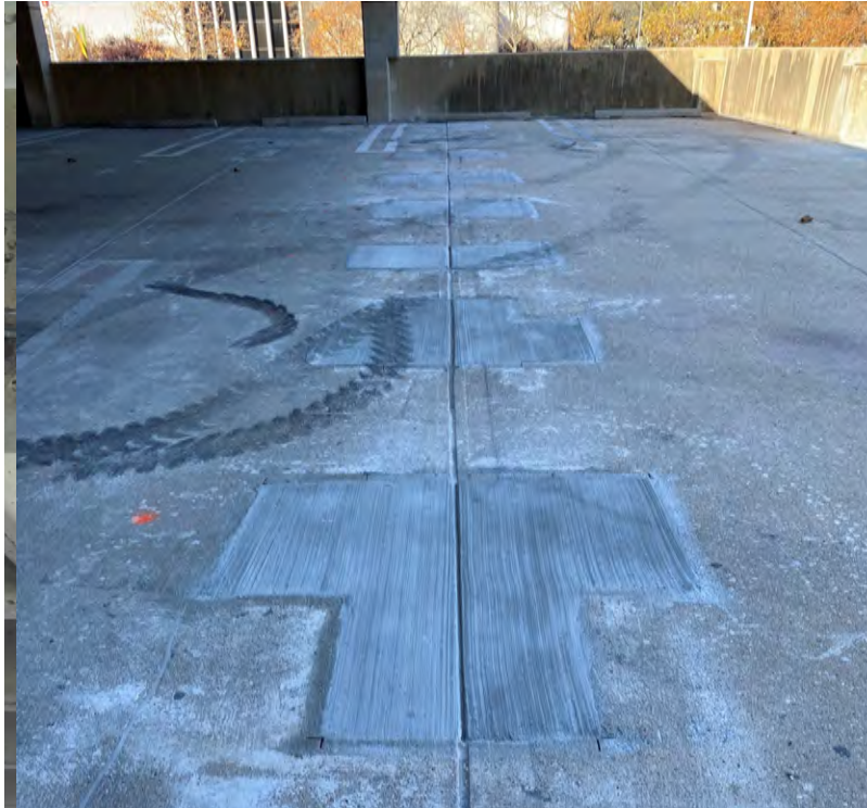
Tee to Tee connections after replacement
