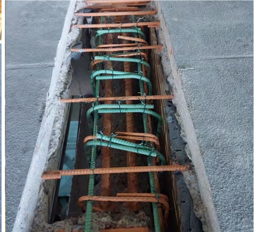
Rebuilding damaged inverted tee beam
