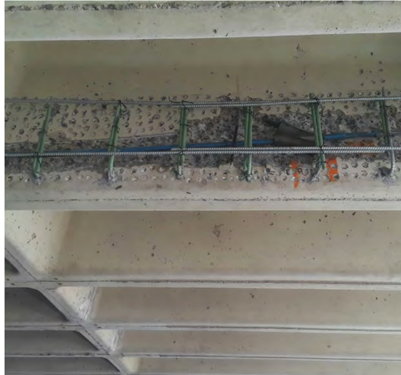
P/T repair at break
