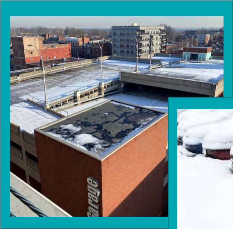
No Live Load - Minimal Snow Load
