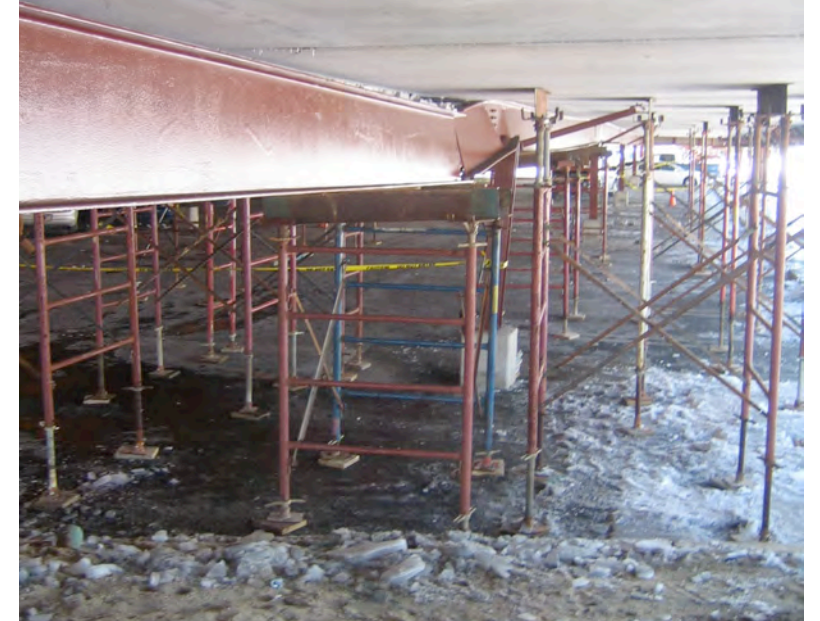
Shoring required for dead and snow loads
