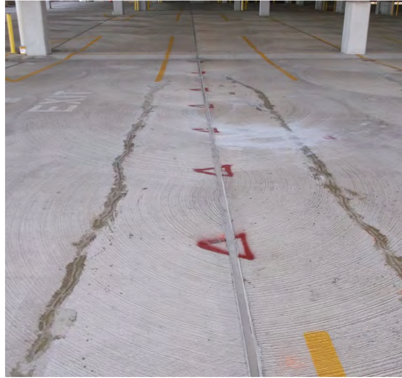
Rewelded tee to tee connections and epoxy injection of cracks
