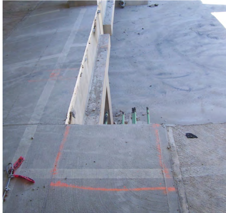
Removed CIP topping over all connections
