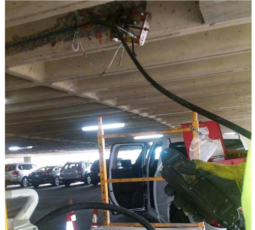
Stressing P/T repair at break
