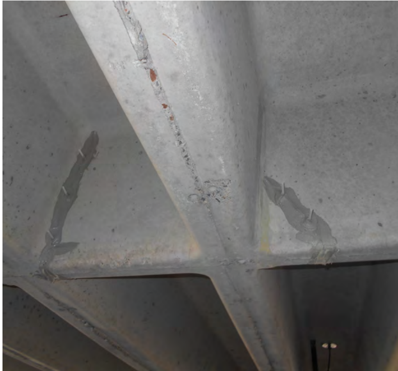
Crack injection in CIP joists
