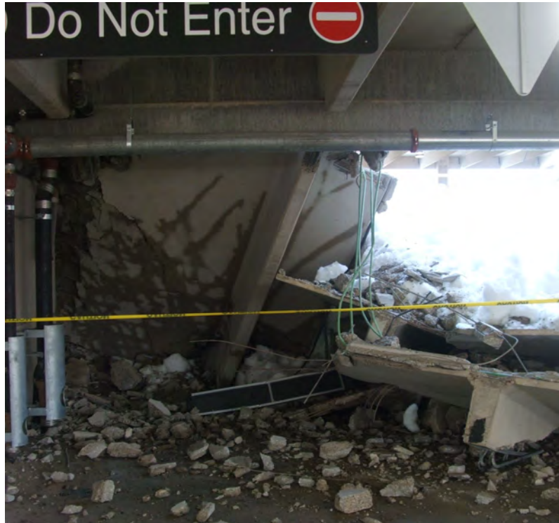
Slab-on-grade failure
