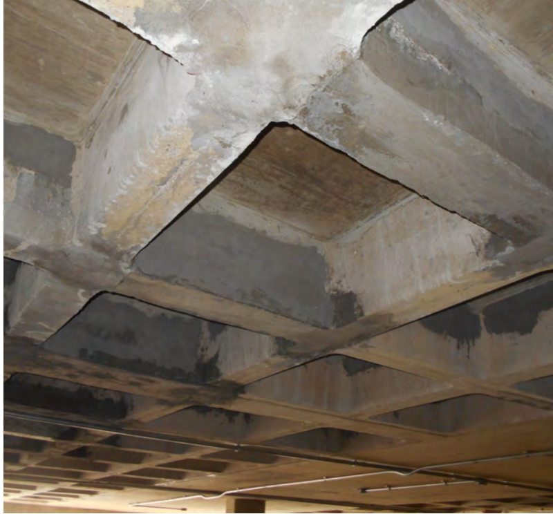
Waffle joist replacement in progress
