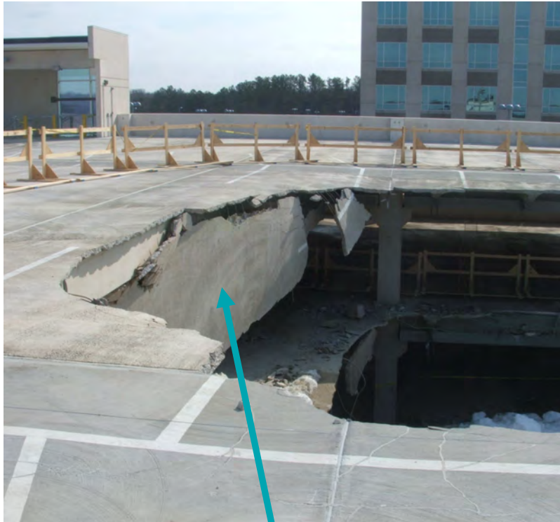
Precast double tee flange and portions of tee stem
