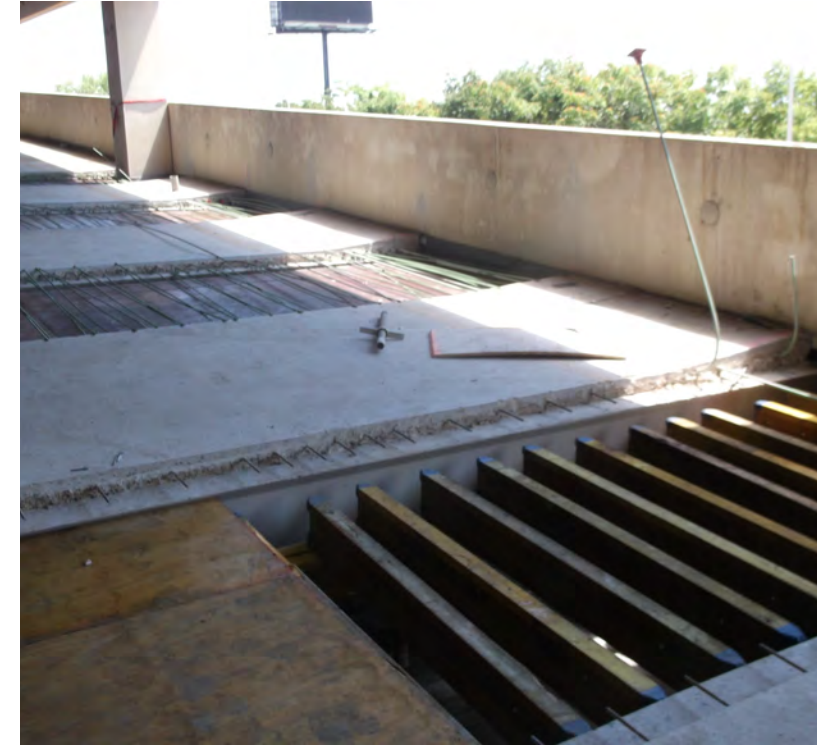
Tee flange replacement in progress
