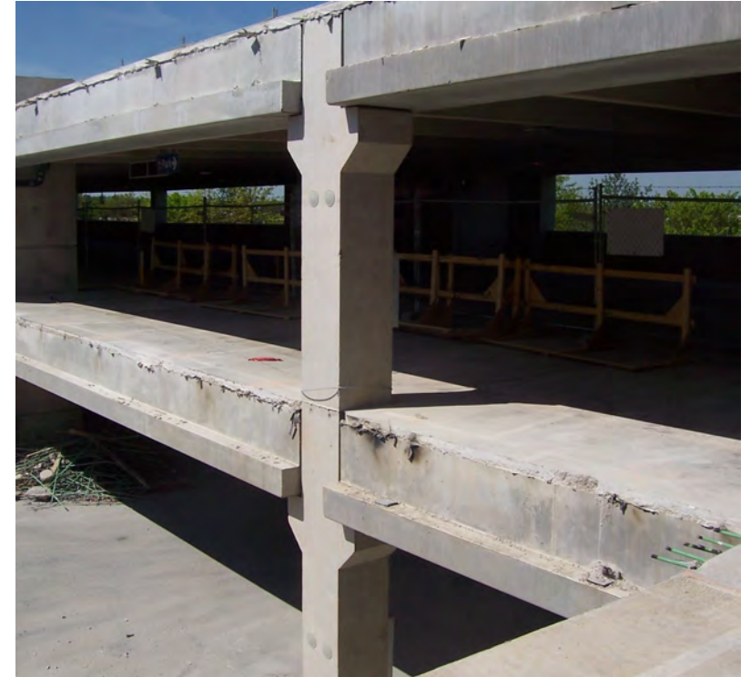
Maintained existing inverted tee beams
