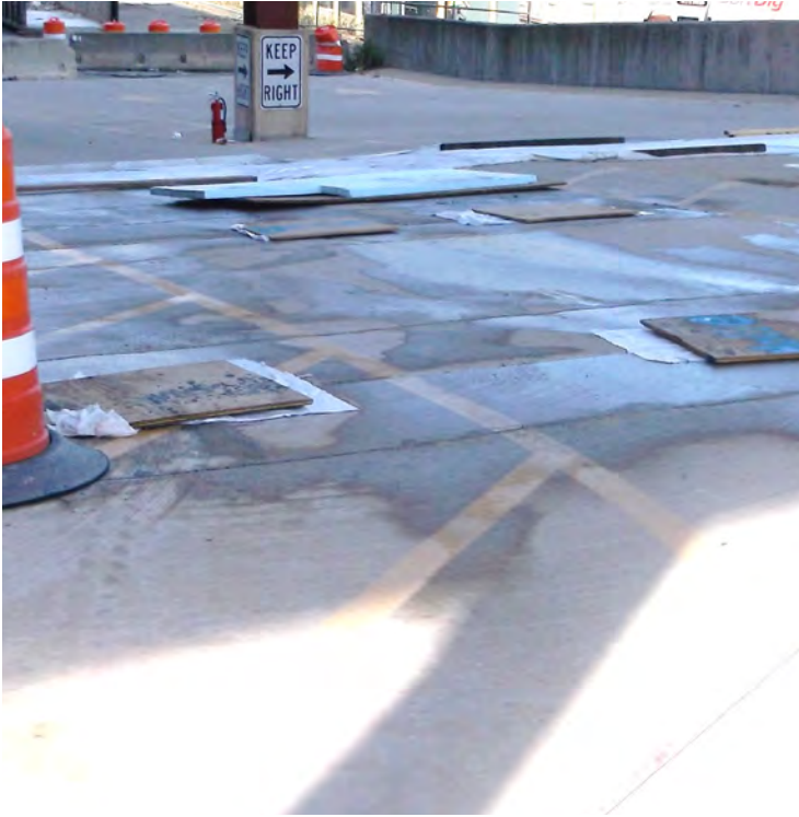
Tee to tee connections during replacement
