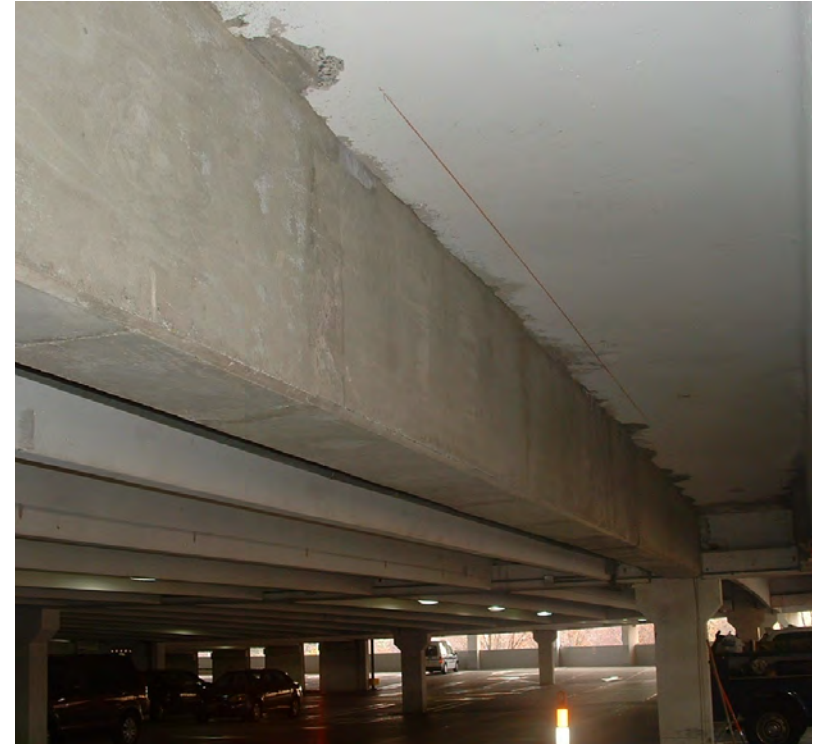
Rebuilt damaged tee stem
