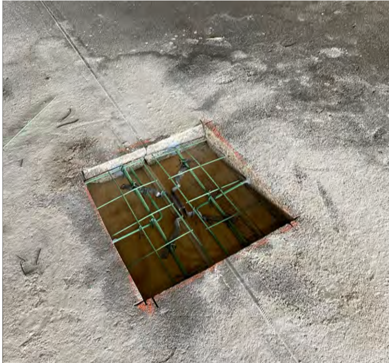
Tee to tee connections during replacement
