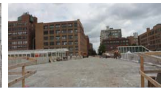
Surface before applying the overlay
