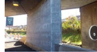
UHPC jacket - Ramp to Pont Victoria under the CN Rail track
