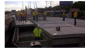
Installation of precast panels
