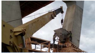
Hoisting and casting from the top of the formwork
