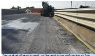
Diamond grinding equipment used to provide grooved running surface
