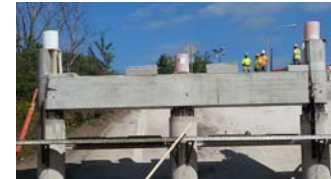
New precast pier cap set on existing columns
