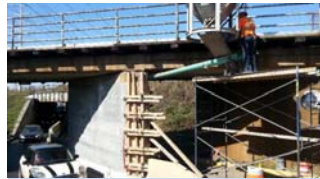
Casting - traffic maintained on adjacent lane
