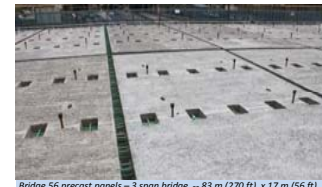
Bridge 56 precast panels - 3 span bridge - 83 m (270 ft) x 17 m (56 ft)
