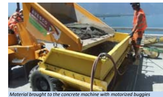
Material brought to the concrete machine with motorized buggies
