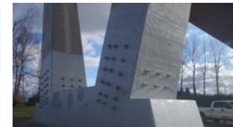
Pier prior to final retrofit
