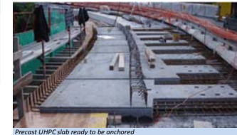
Precast UHPC slab ready to be anchored
