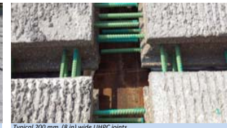
Typical 200 mm (8 in) wide UHPC joints
