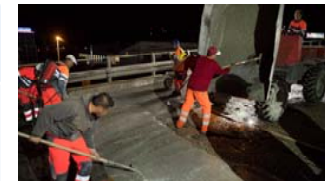
Work performed at night on weekends with traffic back on Mondays
