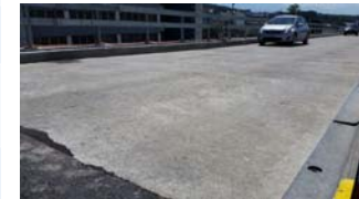
UHPC overlay prior to installation of asphalt layer
