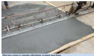
Placing using a simple vibrating screed machine
