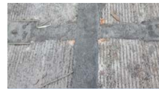
UHPC casting completed
