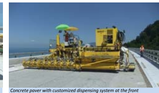
Concrete paver with customized dispensing system at the front
