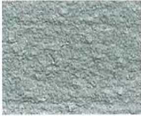
CSP 4 (light scarification)
