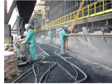
Dry-mix shotcrete Today
