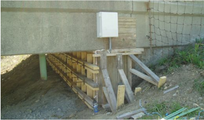
Fig. 6: Formwork and monitoring station prior to pumping SCC
