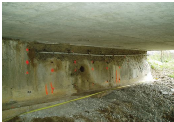
Fig. 4: Concrete spall removal
