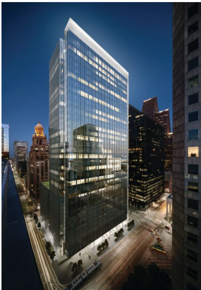
Fig. 1: Bank of America Tower, a 35-story, 750,000-square-foot, Class A office building in Houston features concrete pan formed beams with post-tensioned girders, a mat foundation and concrete core/shear walls. This LEED Platinum certified project demonstrates significantly lower environmental impacts over a typical building and meets the rigorous Life Cycle Assessment (LCA) credit in LEED v4 by using high volume supplementary cementitious material concrete mixes. Image: courtesy of Skanska USA Commercial Development, Inc.
