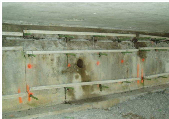
Fig. 5: Dowels and galvanic anodes installed
