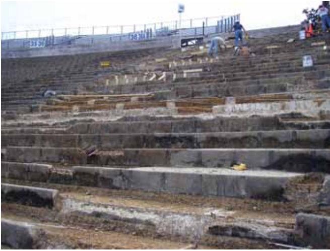
All unsound concrete was removed and new aluminum bench seating was attached to repaired concrete at original lower bowl
