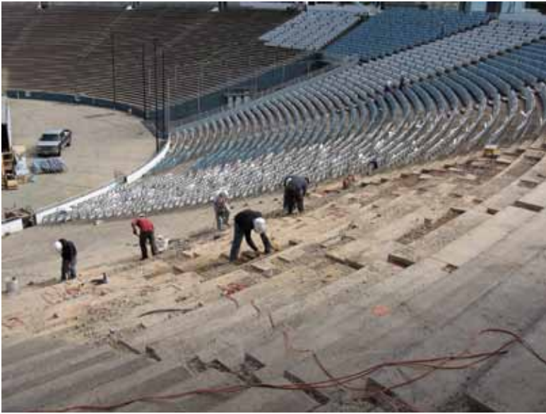
Concrete repair work commenced even before all seating had been removed
