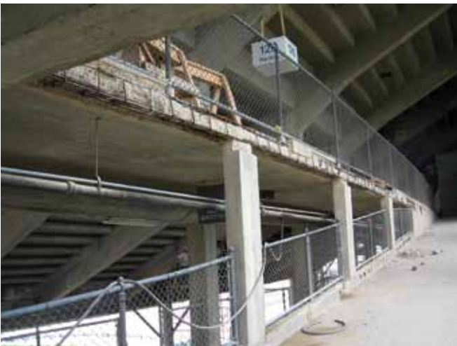
Concourse beam before and after repair
