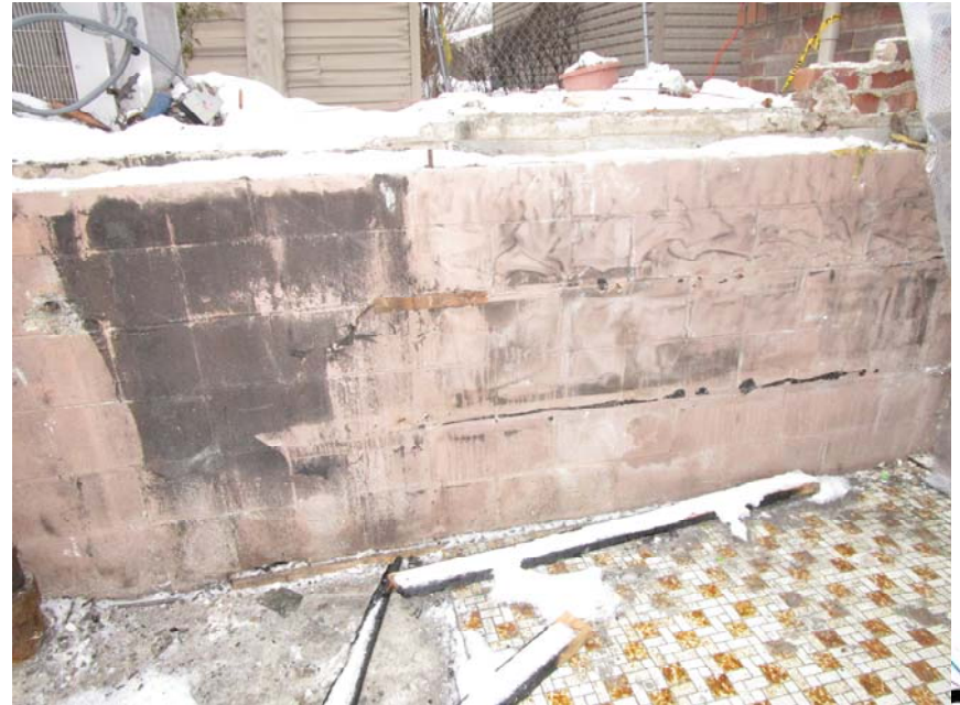
Intact Flooring and Paint
