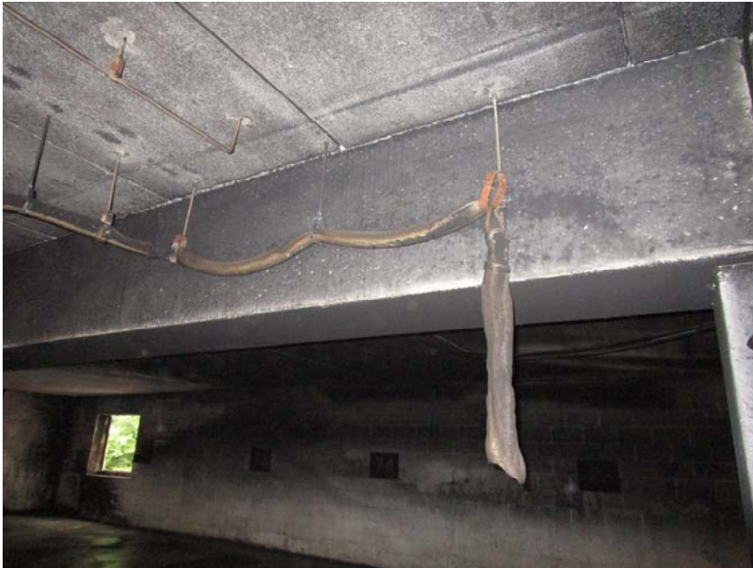
Melted Pipe
