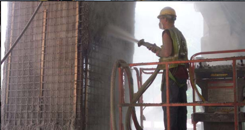
Electrochemical Chloride Extraction
