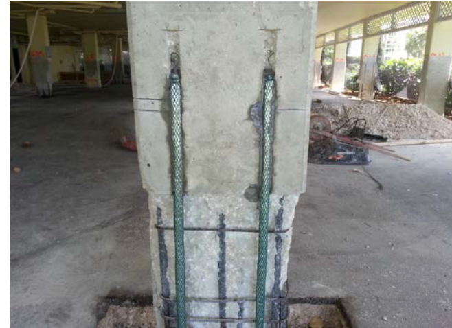
Parking Garage Column Overbuild
