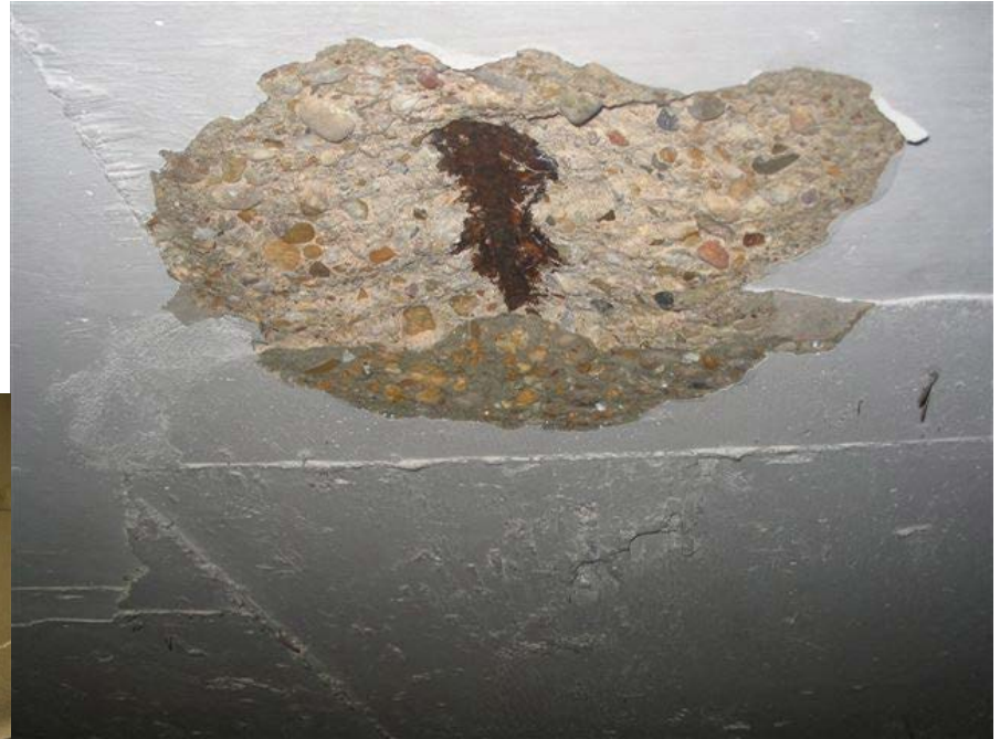
Underside of Parking Deck Washington, DC
