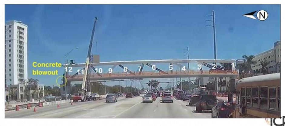
Still image (time stamp 13:46:44:046) from in-vehicle mounted video camera on pickup truck traveling east on SW 8th Street, showing full-width canopy fracture and deck fracture areas at north end (pylon pier), March 15, about 1:46 p.m.
