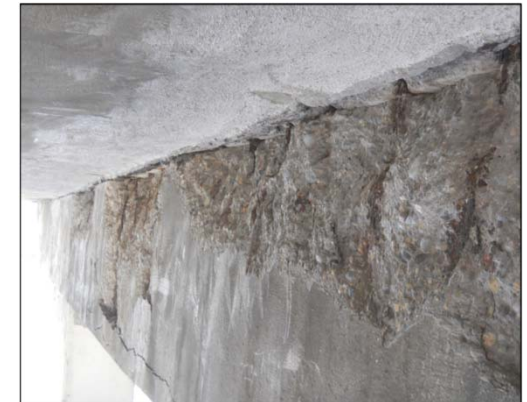
Deterioration of the deck and cap beams
