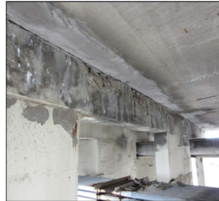
Deterioration of the deck and cap beams
