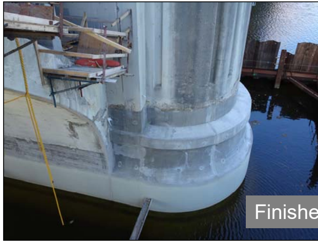
Coffer dams, concrete removals - hydraulic breaker and by detail (chipping/blasting)
