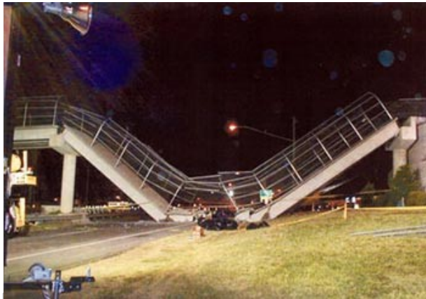
CaCl 2 Grout Lowe's Motor Speedway Bridge Concord, North Carolina --
