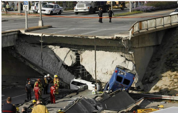
Rebar detailing and installation de la Concorde overpass in Laval Canada — Sept. 30, 2006
