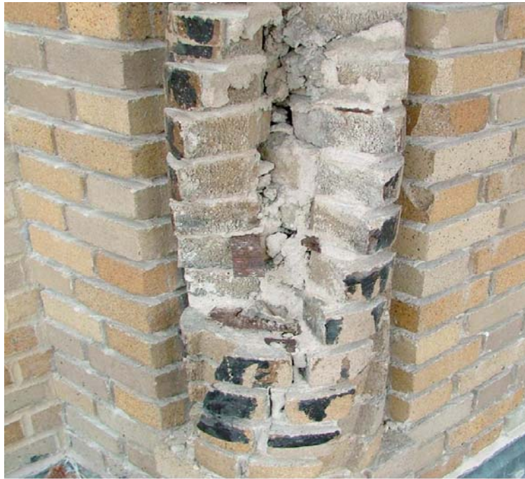
Fig. 3 Special curved roping brick units were replaced after an extensive search for a source
