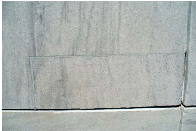
Fig. 6 Marble dutchman repair matches adjacent stone very closely
