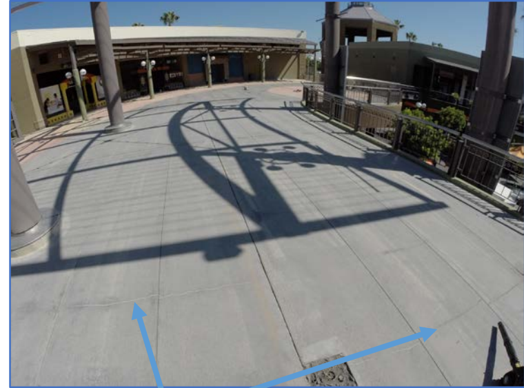
Inadequate Joint Design – Leads to Moving Cracks
