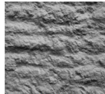
Fig. 6.9: CSP 9 (heavy scarification— rotomilled)
