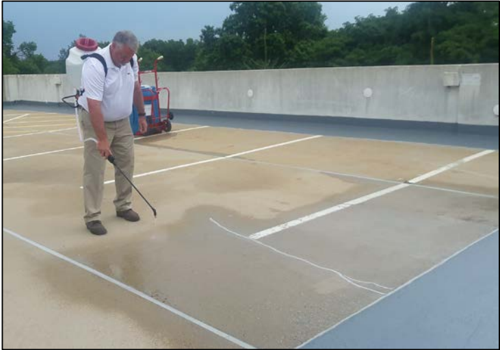
Modified Silica Gel – Spray Applications
