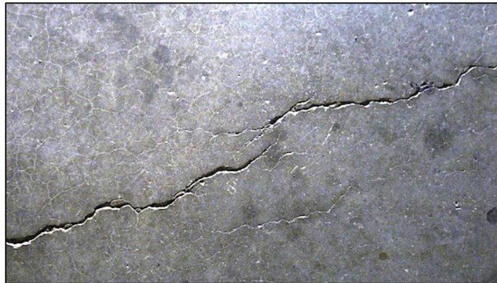
Shrinkage Cracking
