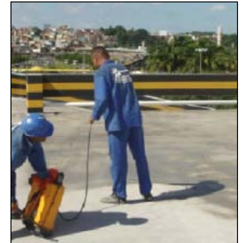
Modified Silica Gel – Spray Applications
