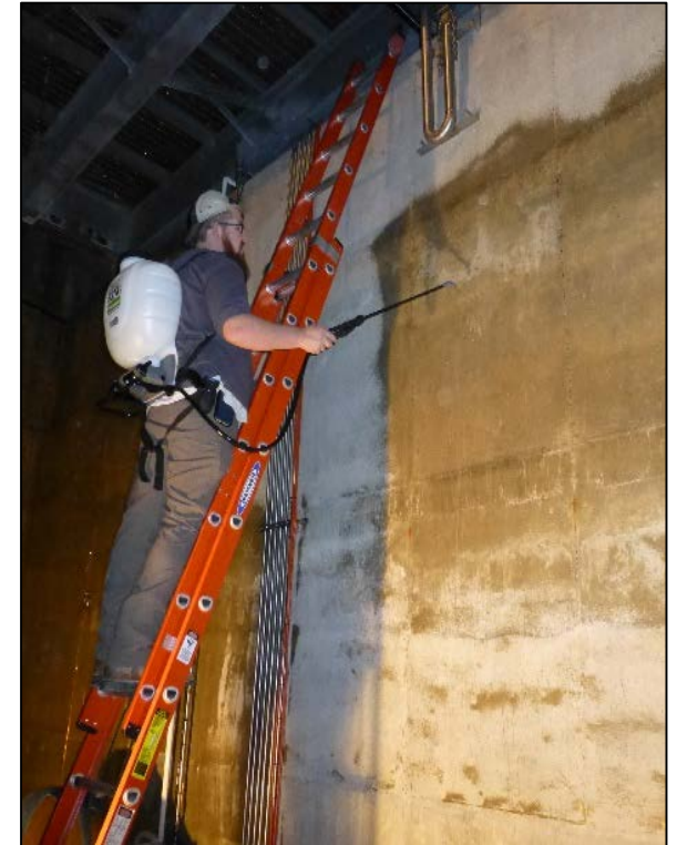
Modified Silica Gel – Spray Application
