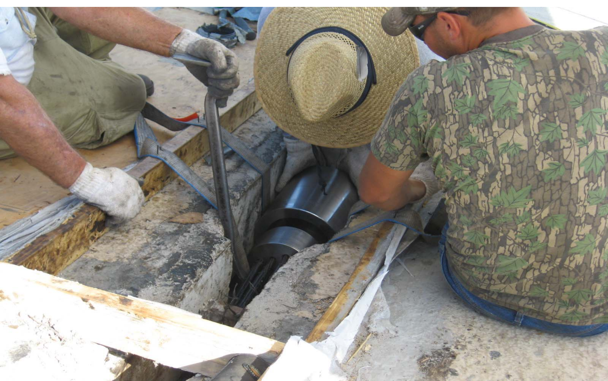
Installation of the New Coupling
