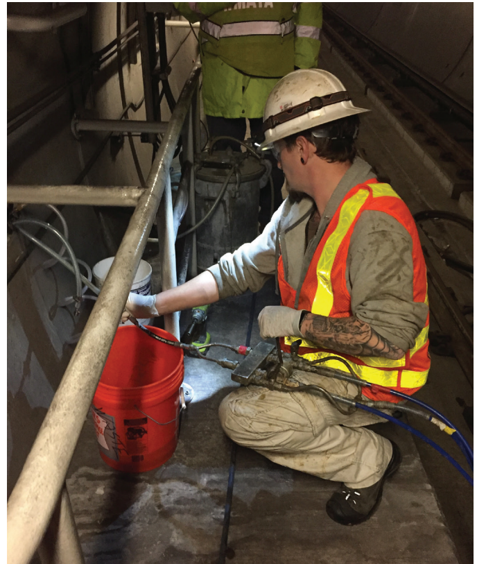
Fig. 2: Two-component chemical injection
