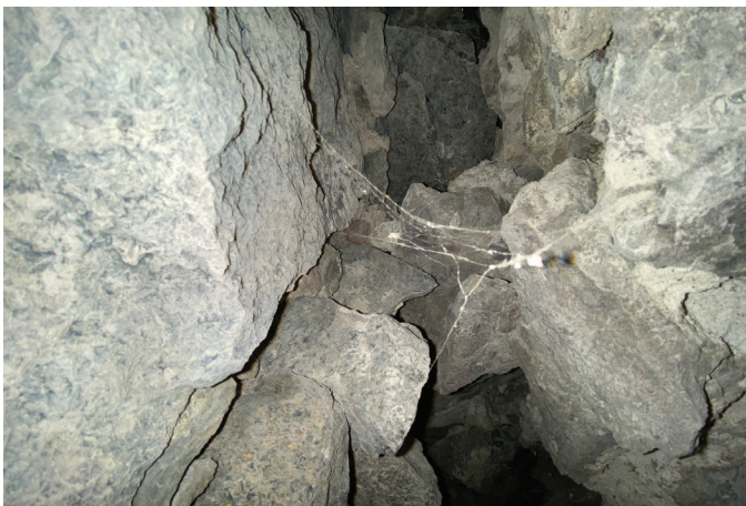
Fig. 2: Image from Inside the Wall Cavity; Exterior Wythe (Left), Back-Up (Right)
