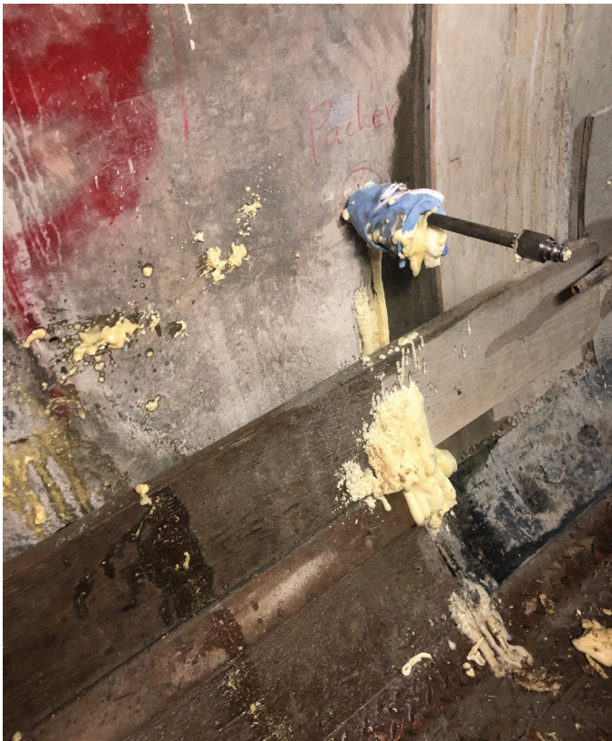
Fig. 5: Polyurethane injection
