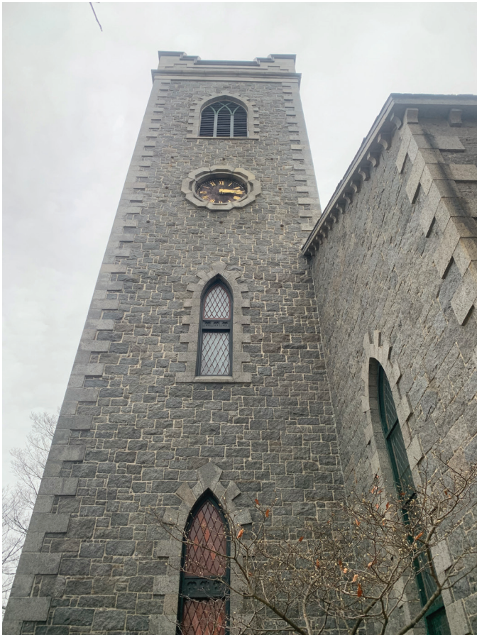
Fig. 1: First Church in Jamaica Plain, Exterior Wall of Tower
