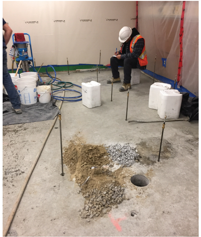
Fig. 4: Grouting for soil stabilization
