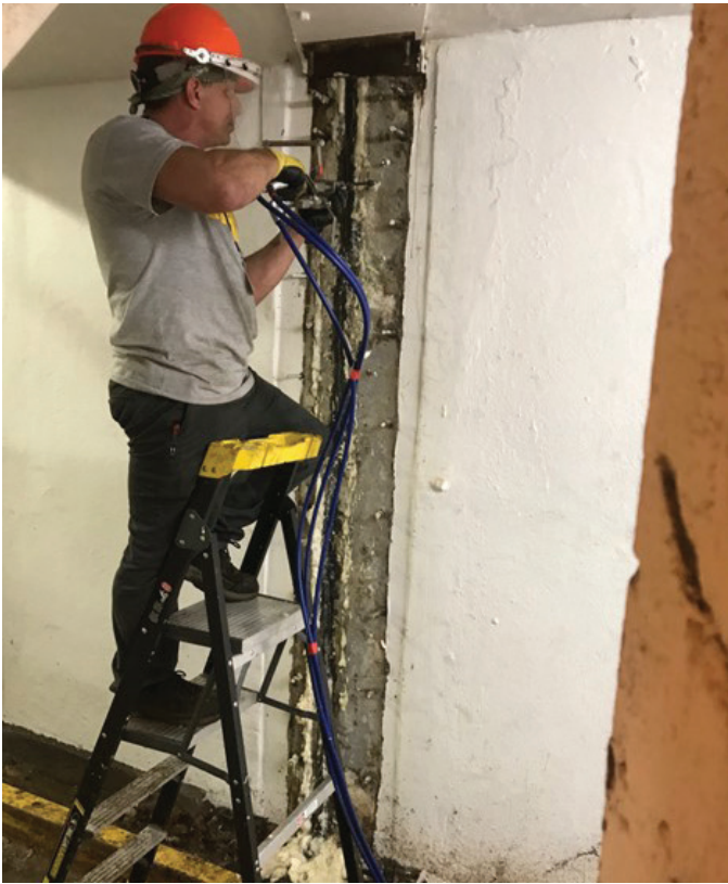
Fig. 3: Three-component chemical injection
