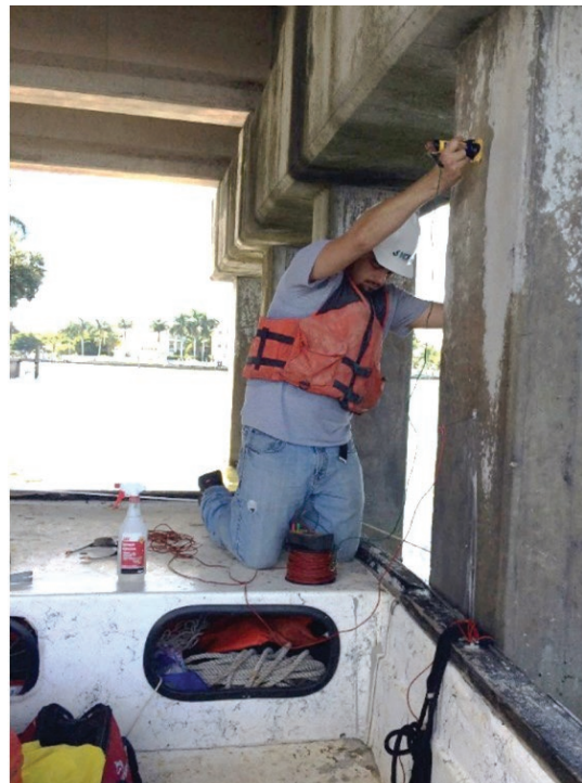
Fig. 4: Corrosion potential testing of prestressed concrete pile
