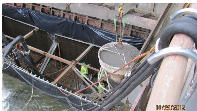
Fig. 5: Transporting concrete down to the repair area via bucket
