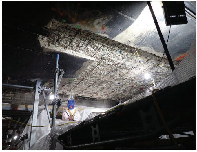
Fig. 11: Overhead concrete repairs on soffit of upper deck during demo.
