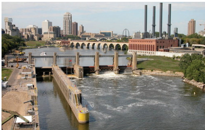
Fig. 1: Lower St. Anthony Falls (LSAF) Lock and Dam
