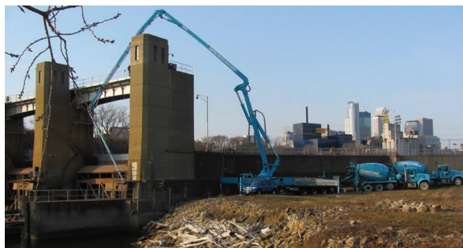
Fig. 6: Transporting concrete down to the repair area via pump truck
