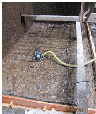
Fig. 3: De-watering of the repair area
