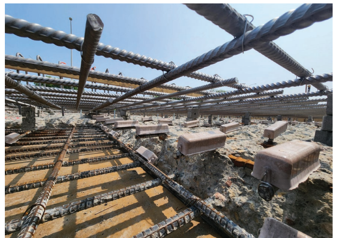
Fig. 2: Galvanic anodes attached to reinforcing steel in bridge deck repair
