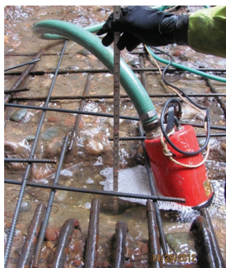
Fig. 4: De-watering of the repair area
