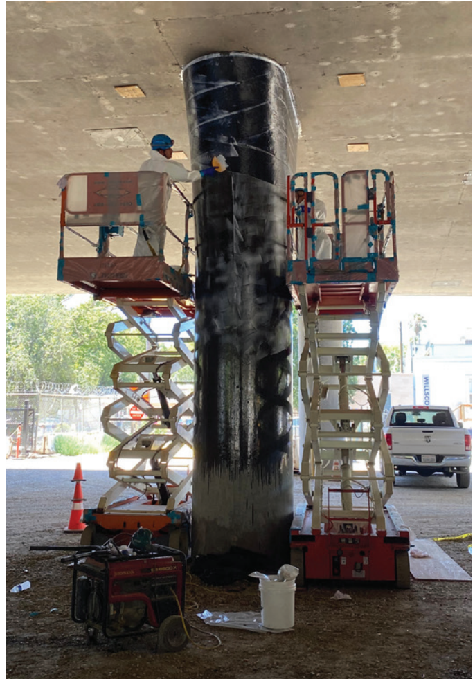
Fig. 4: Applied FRP jacket on the site
