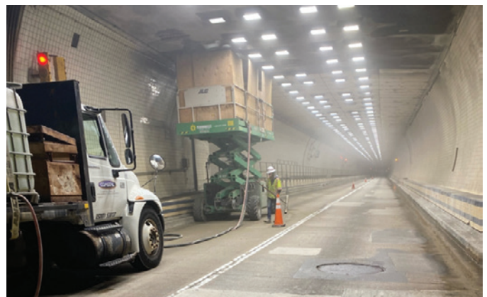
Fig. 3: Placement of Shotcrete in Tunnel
