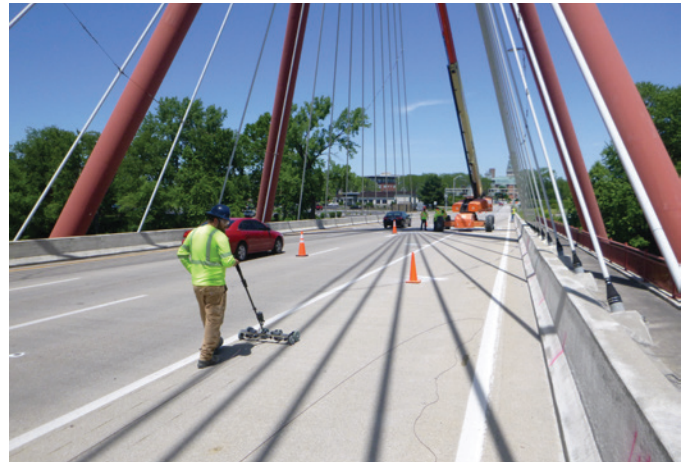
Fig. 5: Half-cell potential survey of a bridge deck
