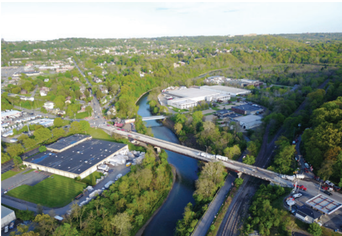
Fig. 6: Pennsylvania Route 60 over Chartiers Creek on the outskirts of Pittsburgh is called the Thornburg Bridge
