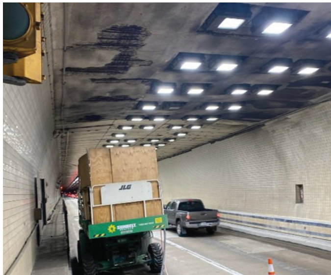
Fig. 4: Prepared Substrate Prior to Shotcrete Installation
