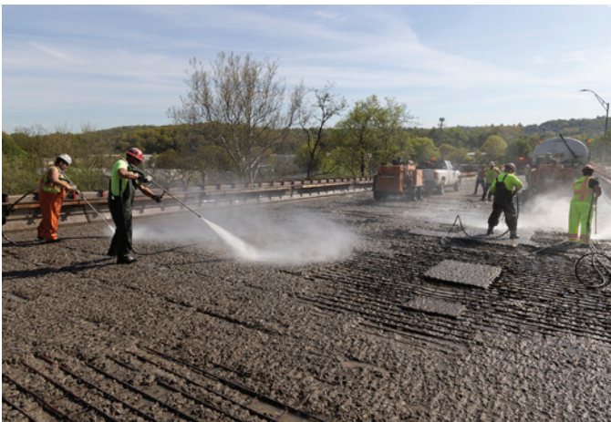
Fig. 3: After removal, the surface was hosed down to remove dust, dirt, and other particles that would compromise the bond. The slurry was vacuumed up and the clean surface covered with polyethylene reflective sheeting to protect it from dripping oil and other contaminants
