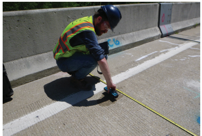
Fig. 6: Surface resistivity survey of a bridge deck
