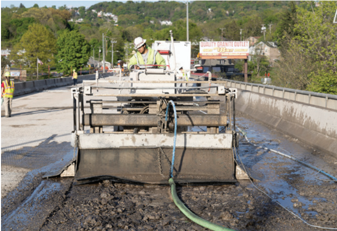
Fig. 2: Hydrodemolition of the Thornburg Bridge. This hydrodemolition robot was calibrated to remove at least an additional 3/4 inch (19 mm) after initial scarification
