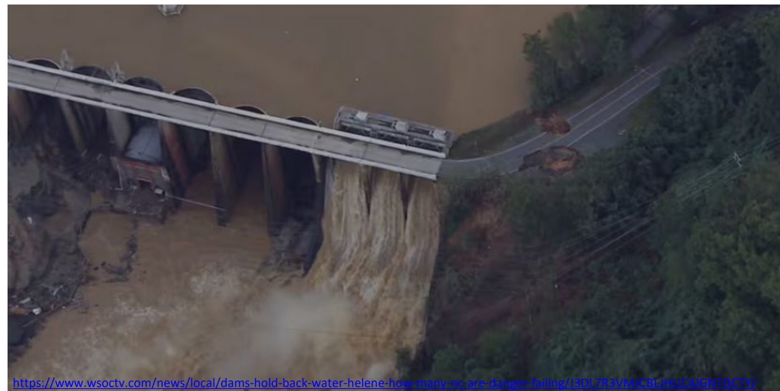
https://www.wsocvtv.com/news/local/dams-hold-back-water-helene-how-many-nc-are-danger-failing/13DL7R3VMJCBLJHUC4JGNTDCTY/ Lake Lure after Hurricane Helene (Sept. 2024)
