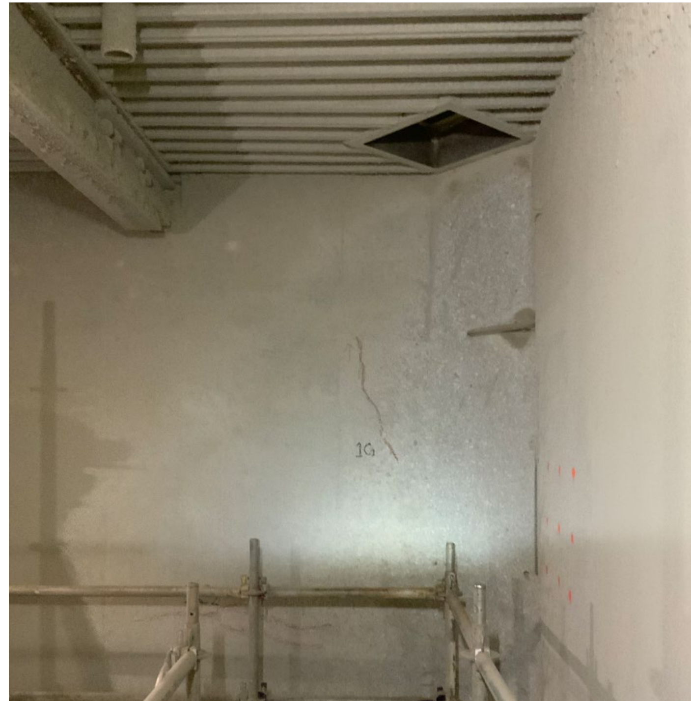
FACING JOINT AT TOP OF SILO
