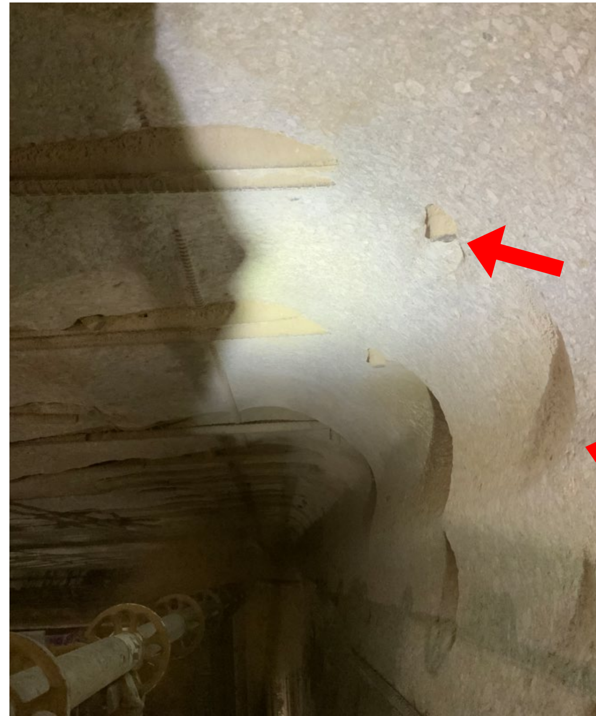
LOOKING DOWN AT JOINT
