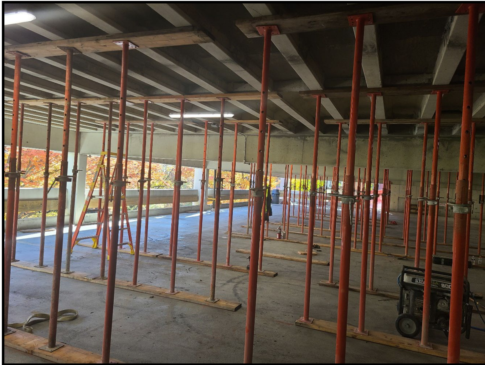
Shoring Posts (Small...)
