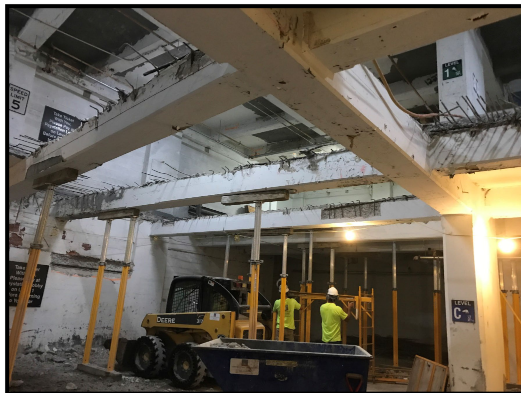
Evaluation for Additional Shoring
