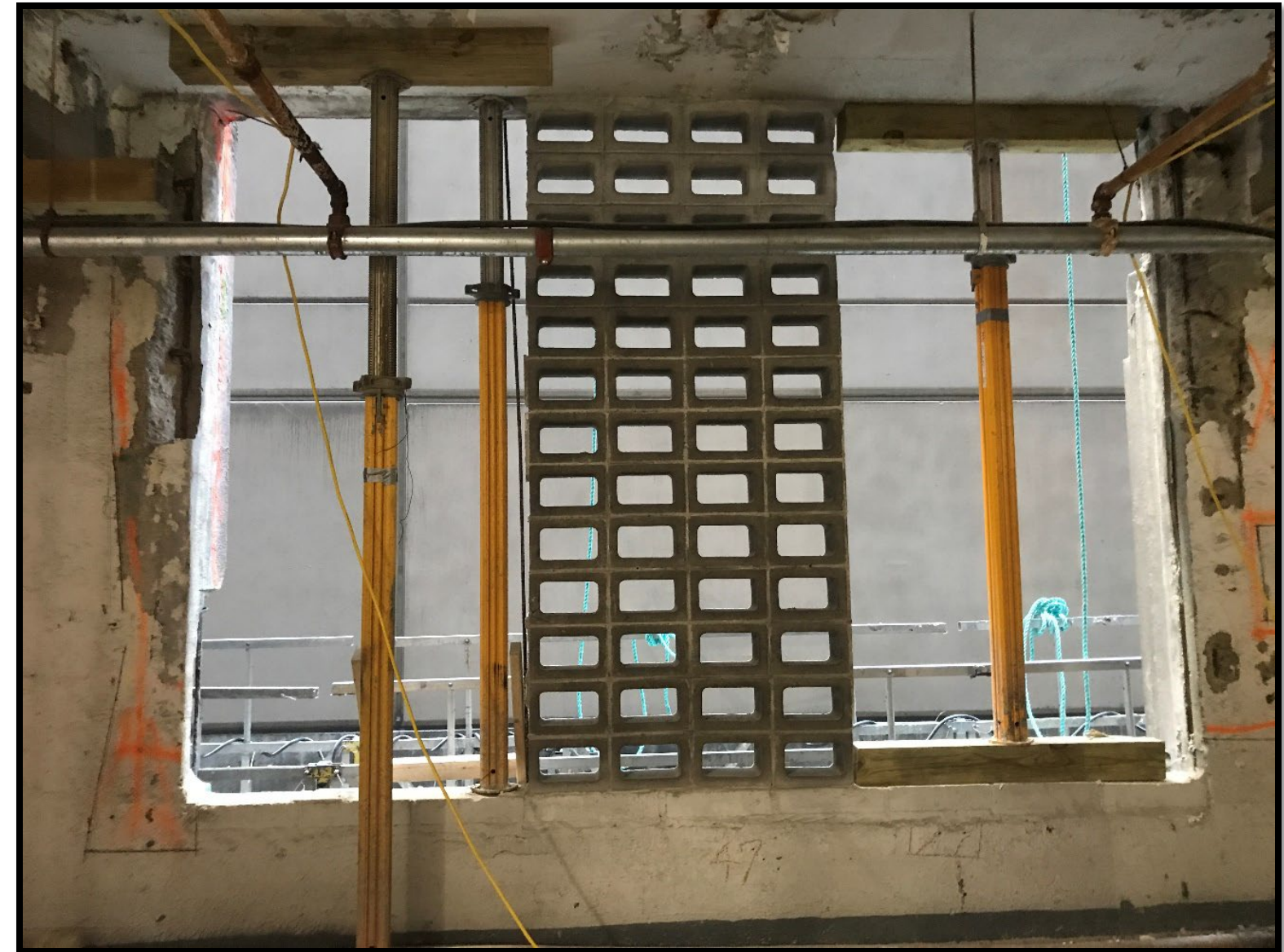
Shoring Posts (and Big!)
