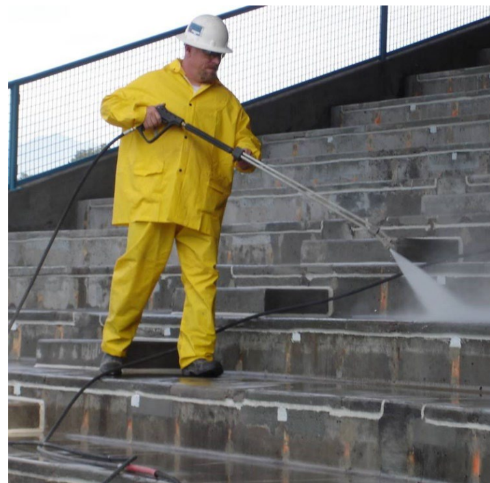
Pressurized Water Cleaning
