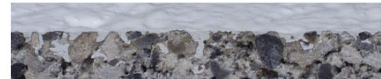
Coating on rough, lightweight concrete
