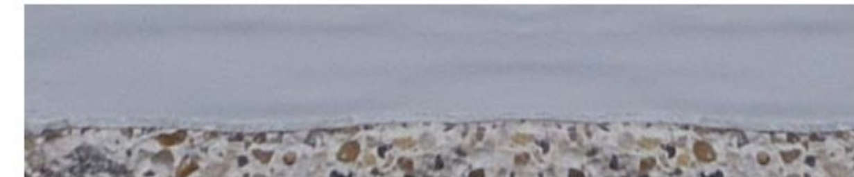
Coating on rough, large aggregate concrete
