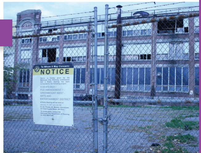
Image 1: The abandoned factory before the renovations
