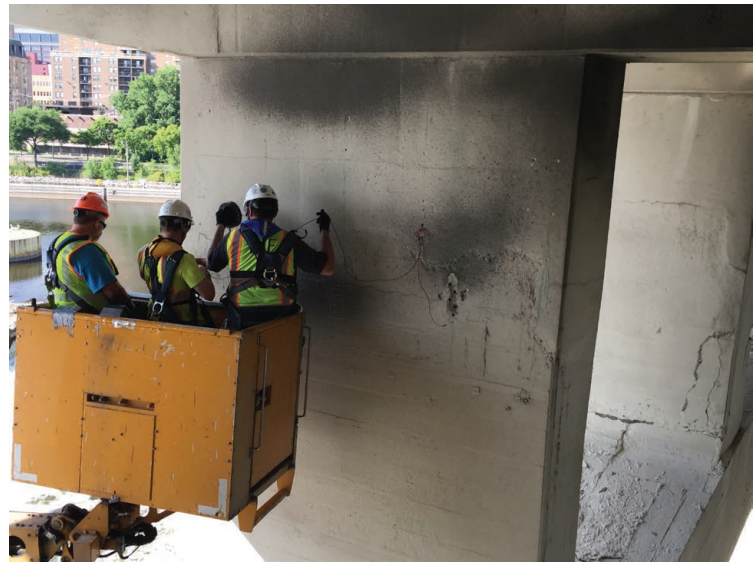
Image 5: Non-destructive testing at spandrel column during bridge inspection and assessment phase
