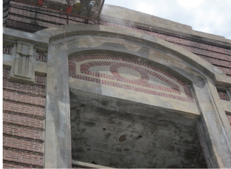
Image 8: Hand-applied mortar in 2014
