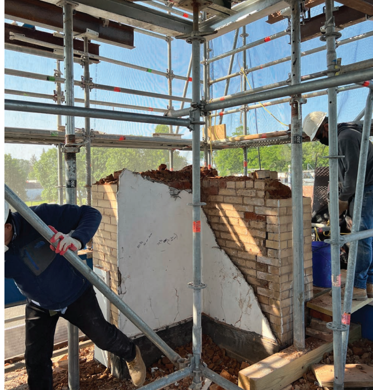
Image 4: Demolition of the tower base with shoring
