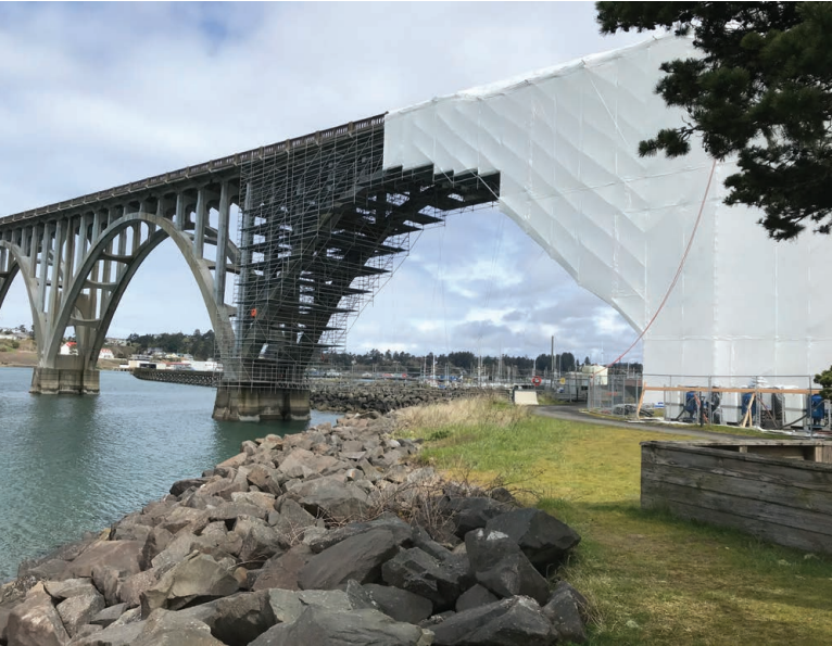
Scaffold with containment
