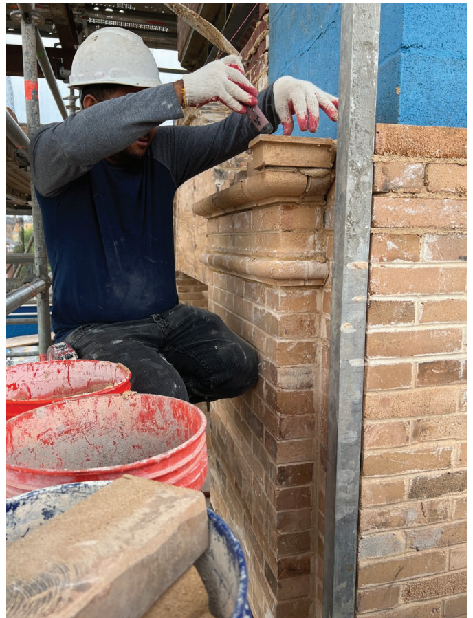
Image 8: Salvaged brick veneer installation
