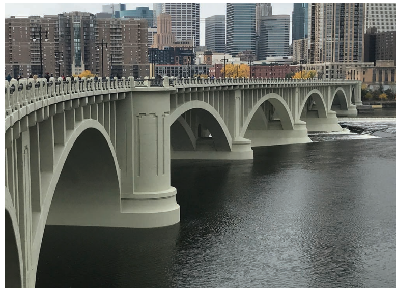
Image 14: "After" photograph along upstream of bridge, showing repaired arches and pier bases with new coating, along with replaced columns, cap beams, and railings above
