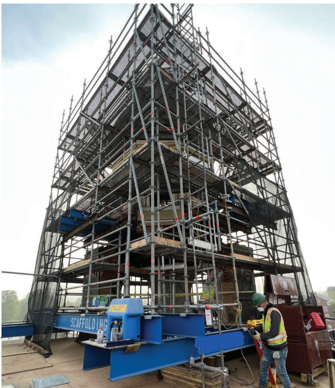
Image 6: Suspension of the upper two-thirds during reconstruction of the base
