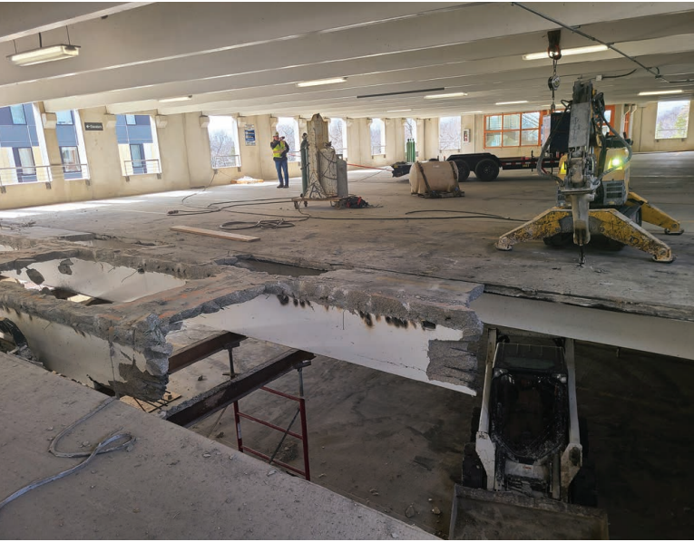
Image 6: Remote controlled demolition
