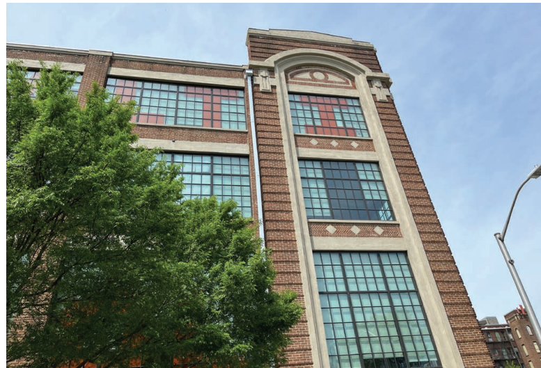
Image 9: Façade of building 10 years later
