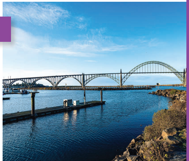
Yaquina Bay Bridge
