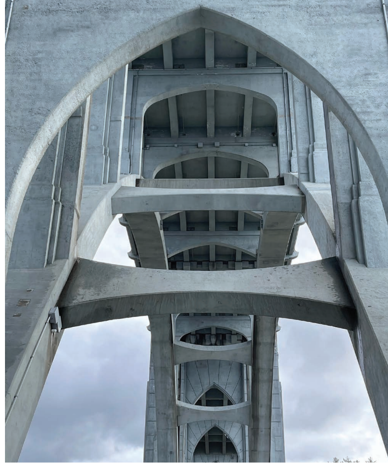
Completed cathodic protection installation
