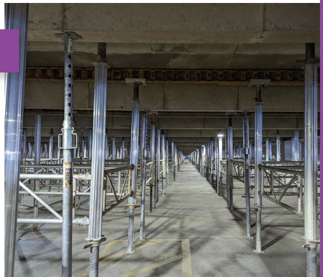
Typical shoring layout for slab strengthening slot installation
