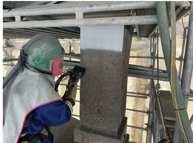
Metalizing on a properly prepared concrete surface
