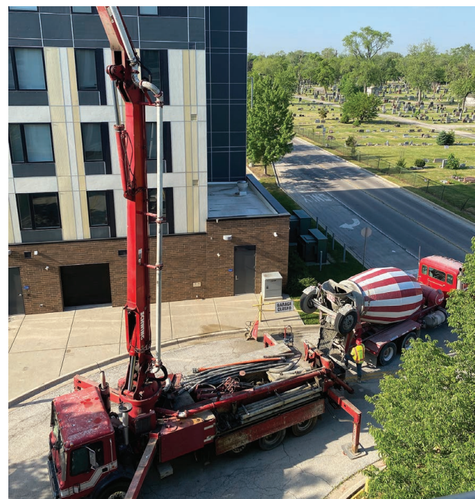
Image 5: Pump truck positioned to pump through opening
