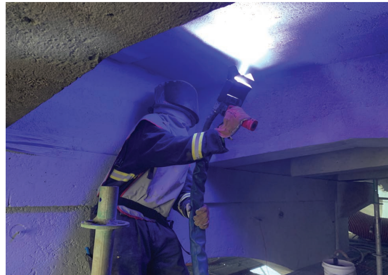
Installing thermally sprayed ICCP system
