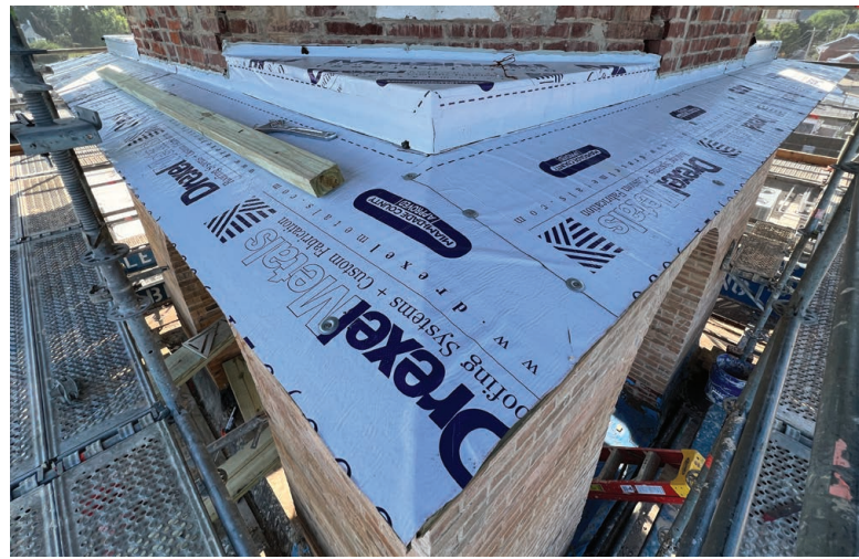
Image 7: Waterproofing and flashing materials installed
