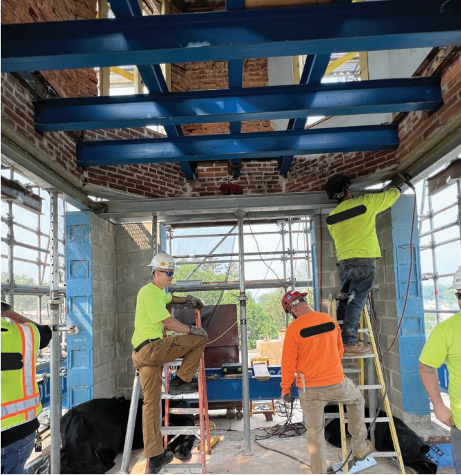
Image 5: Tower base reconstruction with structural steel installed
