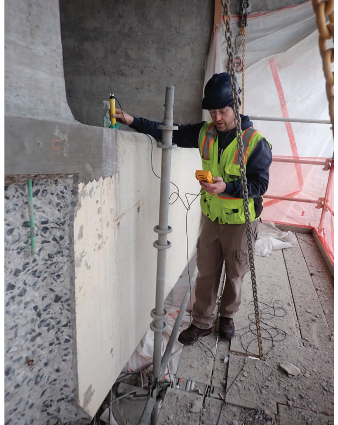
Image 10: Half-cell potential testing during construction
