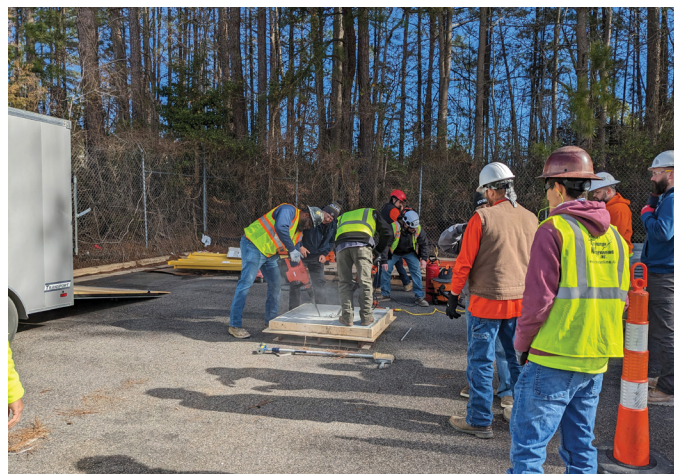
Training on Mock-Up Slabs – Raleigh, NC
