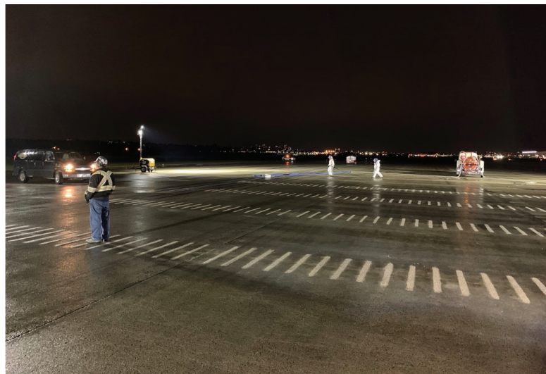
Fig. 6: Complete retrofitted joints
