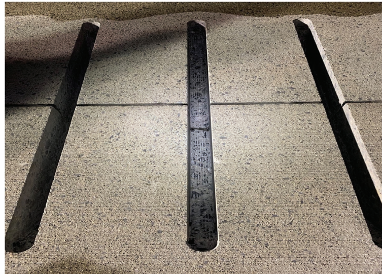
Fig. 4: Initial concrete removal from cuts
