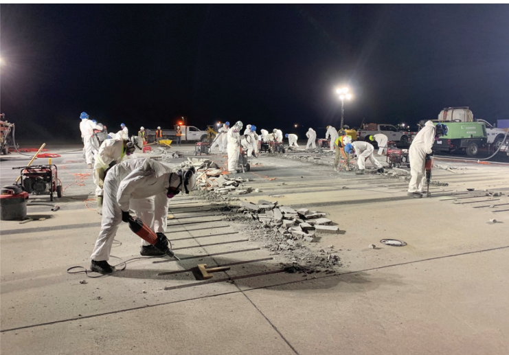
Fig. 5: Slot preparation for dowels and backfill
