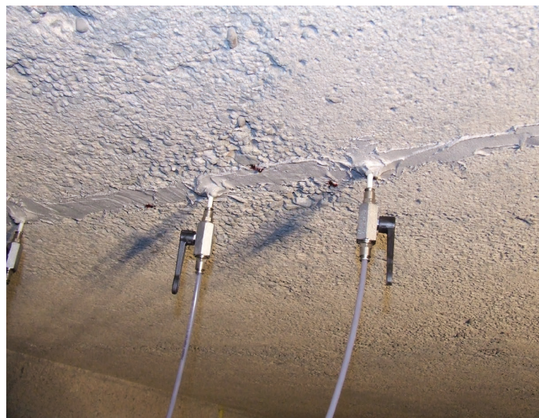
Fig. 1: Example of manifold epoxy injection
