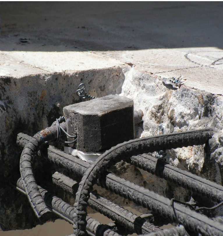
Fig. 8: Galvanic anodes protect repairs against "Halo Effect Corrosion"
