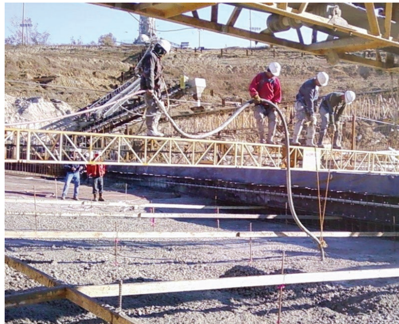
Fig. 2: Original 2011 installation of the overlay at the Lilly Bayou Control Structure
