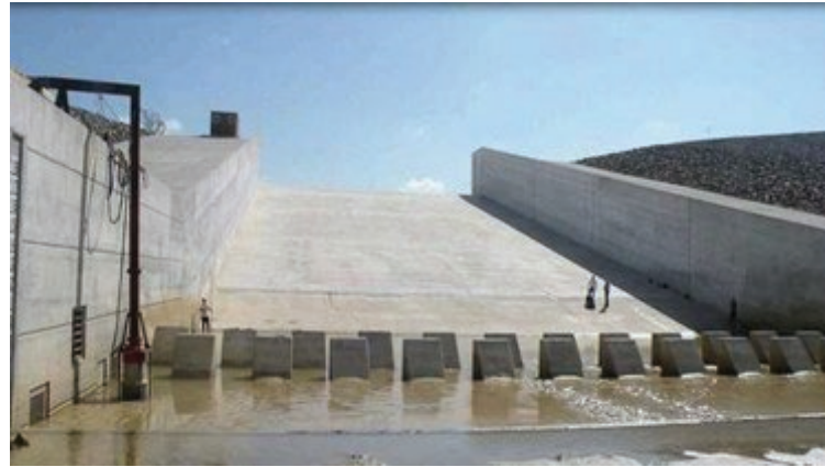
Fig. 5: Degree of slope in the spillway
