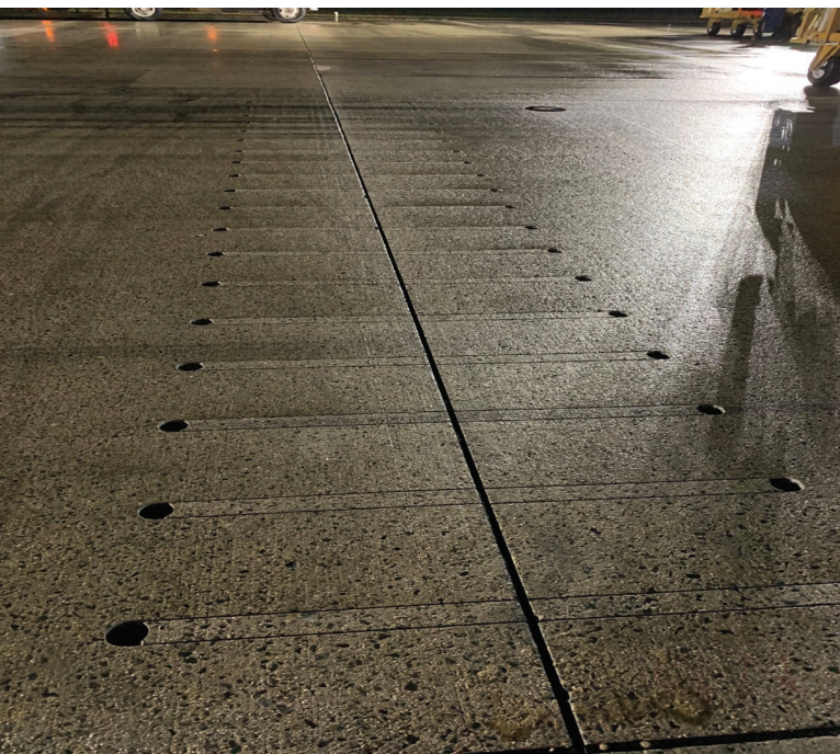
Fig. 3: Precision doweling and cuts performed
