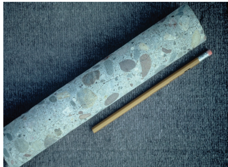
Fig. 2: Cored sample of a full depth crack
