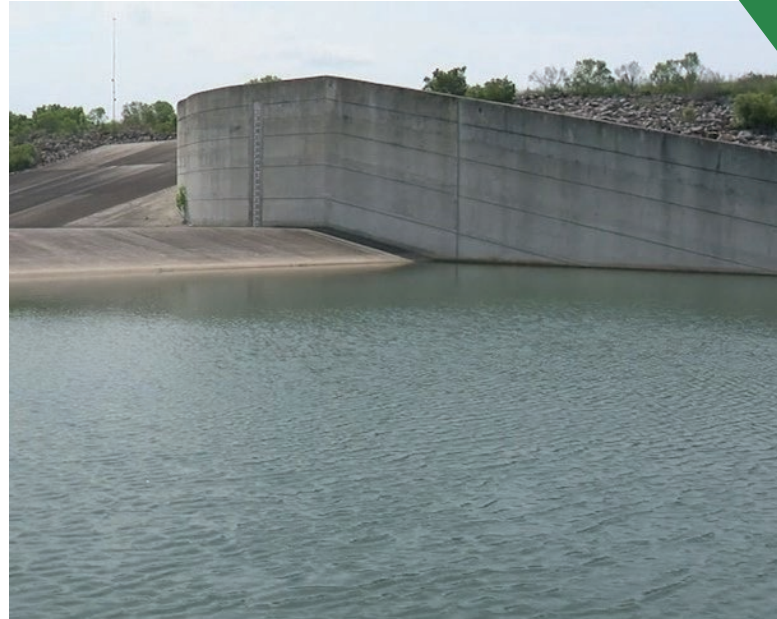
Fig. 1: Lilly Bayou Control Structure
