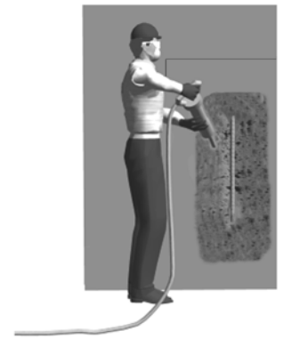
Unsound concrete removed with 15-lb chipping hammer. Hammers larger than a 15-lb class may cause damage to substrate and reinforcement.
