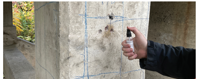
Fig. 8a: Carbonation Field Test—spray-applied pH indicator (phenolphthalein) at drill holes of incremental depths
