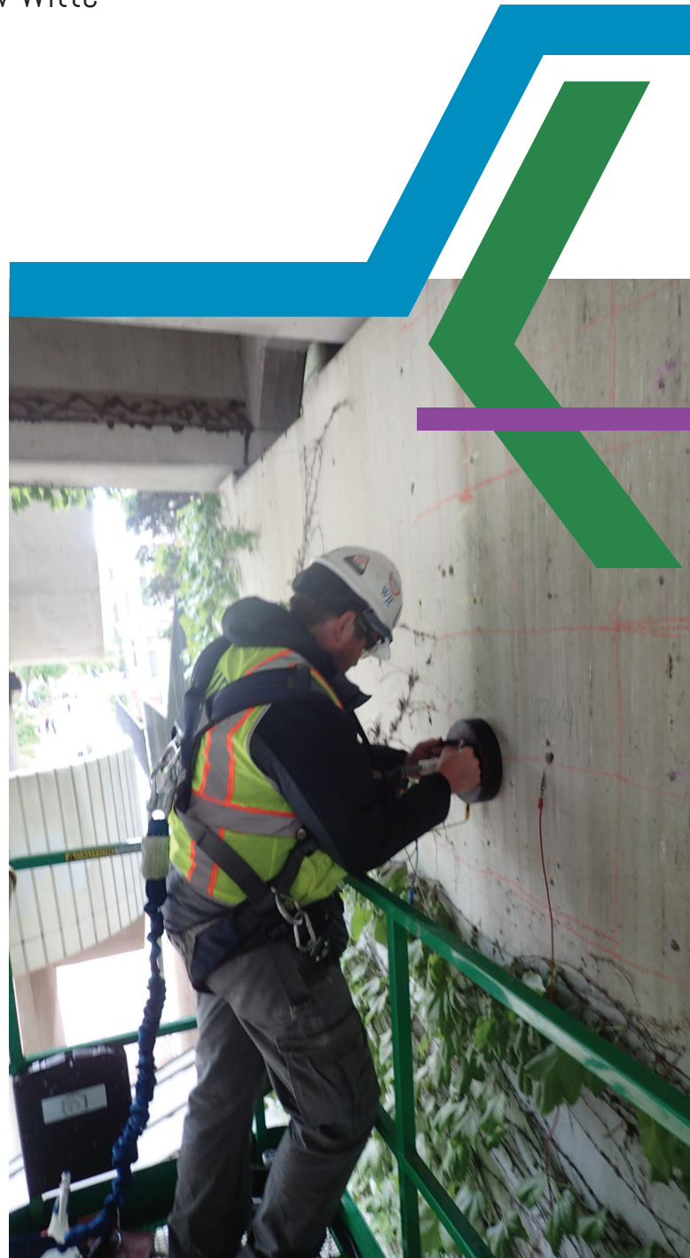
Corrosion rate testing of reinforced concrete
