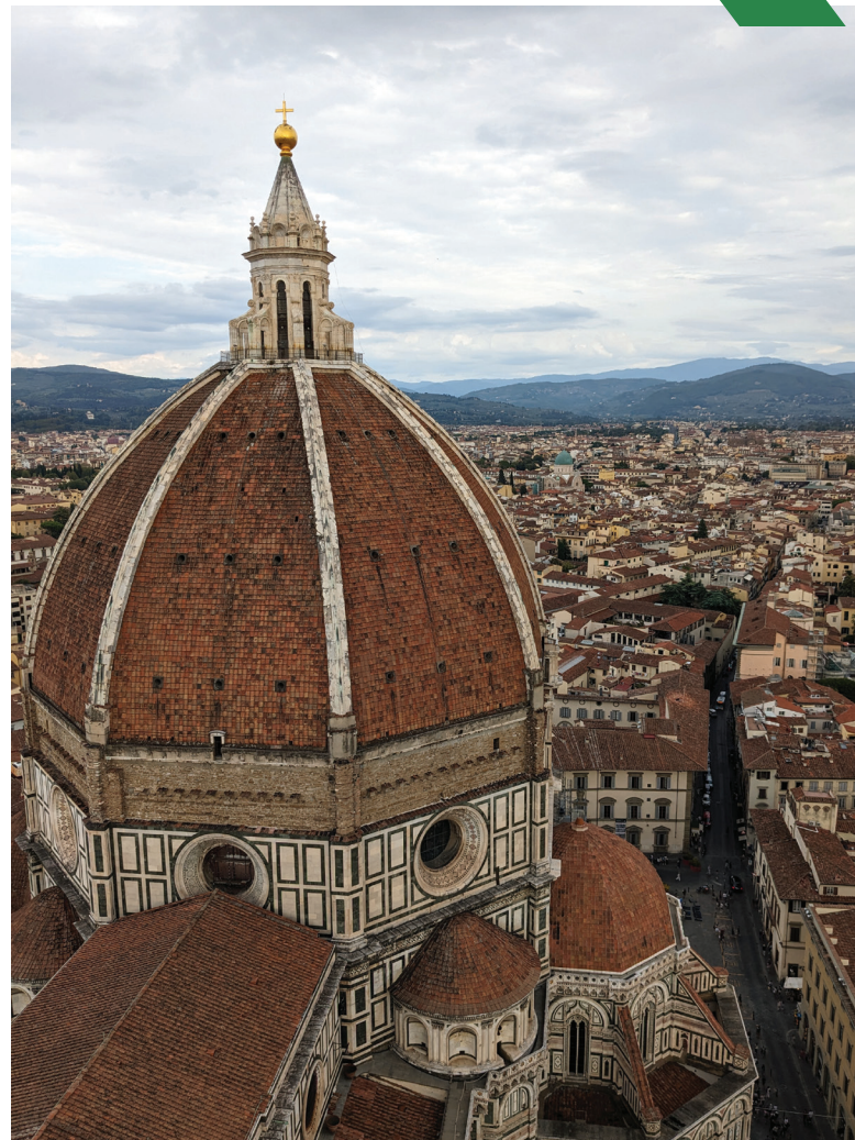
Fig. 1: Brunelleschi's Dome in Florence, Italy (Duomo di Firenze) (Image courtesy of the author)
