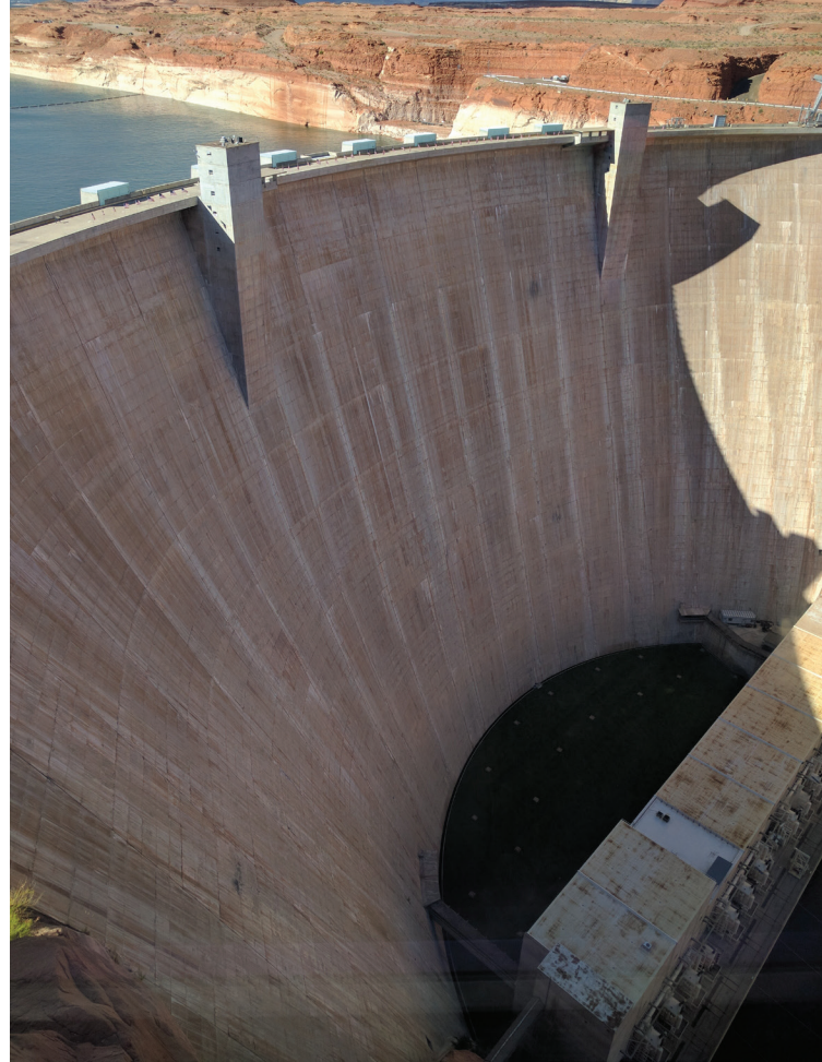
Fig. 2: Glen Canyon Dam, a concrete arch-gravity dam built in the 1960s on the Colorado River, impounds Lake Powell and provides flood control, irrigation, and hydroelectricity in the American West (image courtesy of the author) 2
