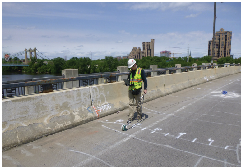
Fig. 5a: Half-cell survey method — rolling half-cell survey of bridge deck
