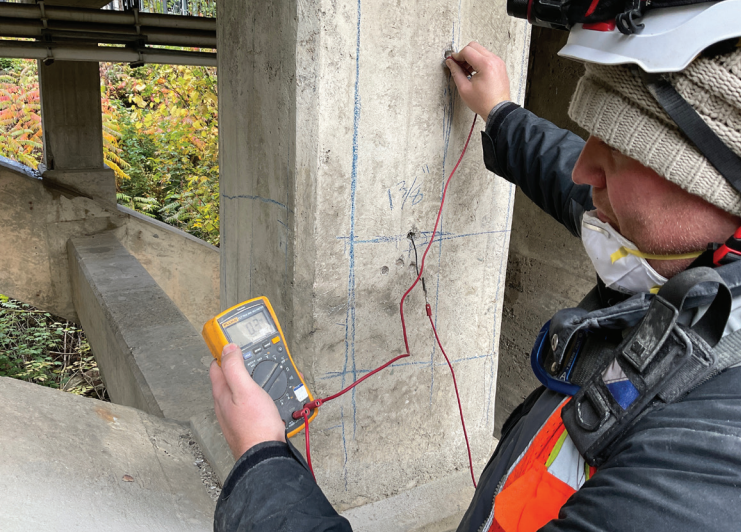
Fig. 4: Rebar continuity verification
